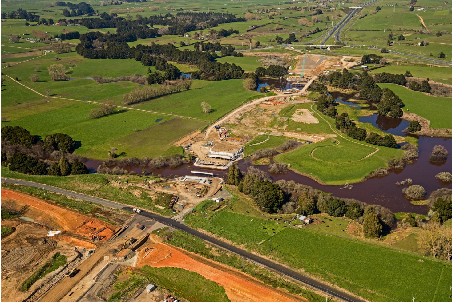
Photo 7: Mangatoketoke and Komakarua Stream bridge sites following storm event in July 2016, where water overtopped the clothed embankments and swamped the crane platforms. In-house control and manufacture of precast elements enabled successful sequencing in areas where high water levels meant access delays. Additional photos show extent of ground surface flooding at the northern end of the site
