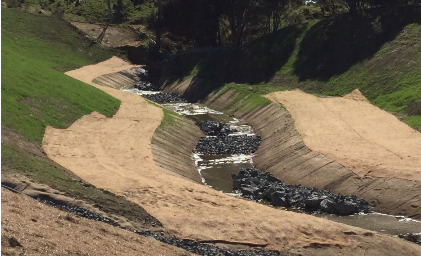
Photo 5: (August 2016) Example of stream diversion works, stream diversion 14, a reconstructed meandering stream to mirror the existing conditions of the relocated waterway.
