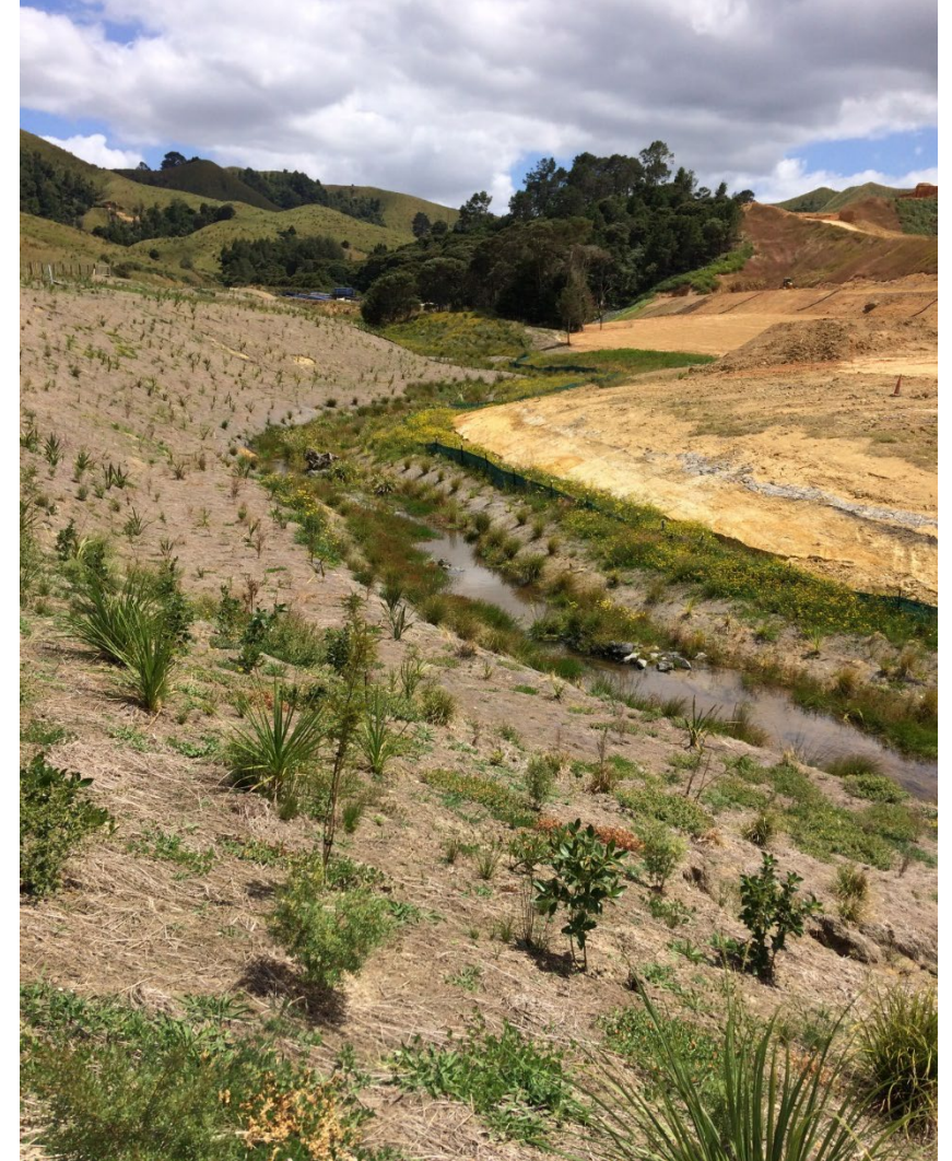
Photo 5: (August 2016) Example of stream diversion works, stream diversion 14, a reconstructed meandering stream to mirror the existing conditions of the relocated waterway.
