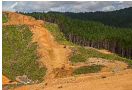
Building access in Central North
