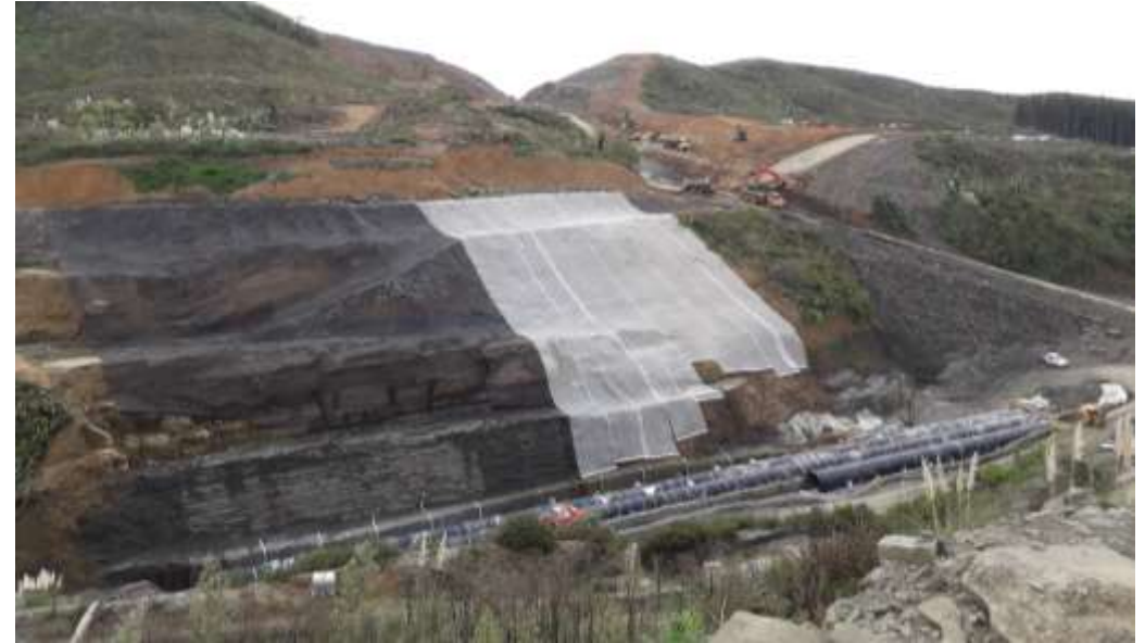
CN8A following slip removal & culvert installation
