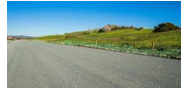
Pavement preparation underway New Zealand Government
