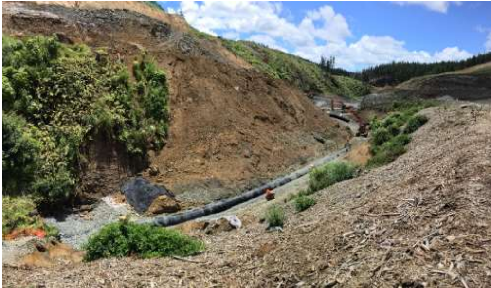
Emergency stream diversion installed for incoming weather event
