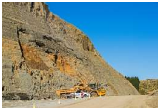
Rock batter in Central North
