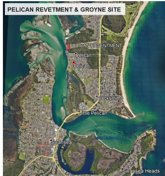
Figure 2: Pelican revetment site
