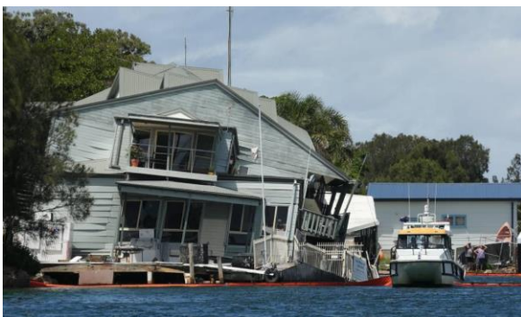
Figure 6: Pelican at time of building collapse (building removed by others) – image printed in Newcastle Herald taken by Simone De Peak
