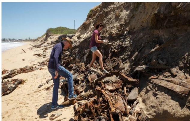
Figure 8: Source Newcastle Herald – Stockton community members inspecting degraded landfill site exposed by erosion
