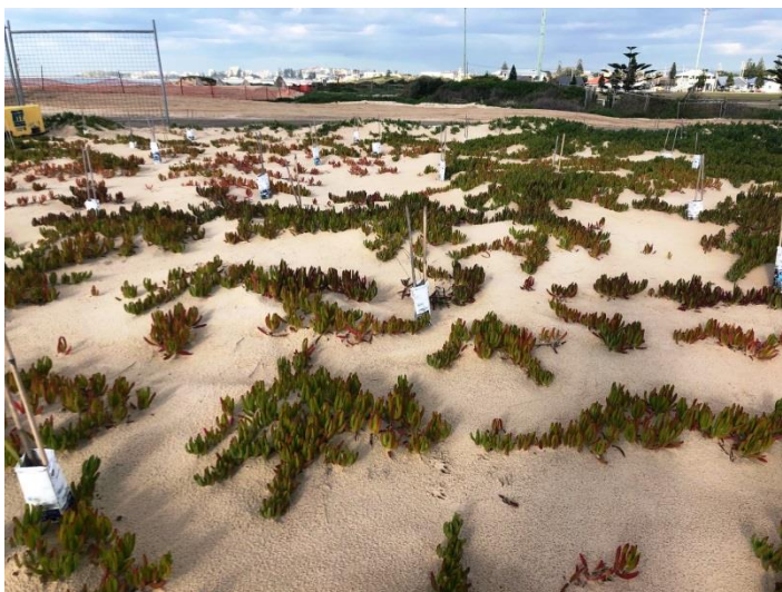
Figure 5: Progressive revegetation undertaken by Hunter Water on decontaminated surface of landfill site – note exclusion fencing in background – maintained throughout the construction process.
