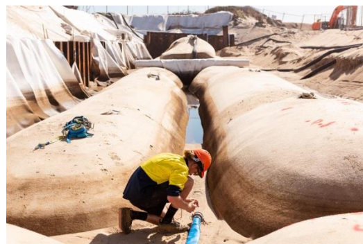
Figure 22: The joys of becoming an expert. Mega Container implementation at Stockton, again, & again & again.
