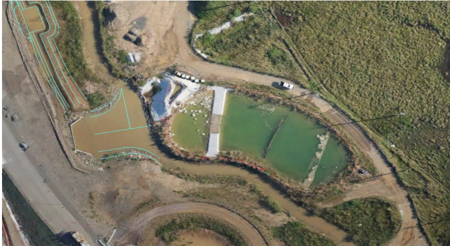
Figure 8 A modified turkey nest arrangement at the Caloundra Road interchange, shown here from above, captures and treats all sub-catchments within the interchange work area.
