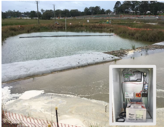
Figure 9 A ground perspective of the retrofitted turkey nest and inset showing the inside of the solar powered in-line dosing unit.
