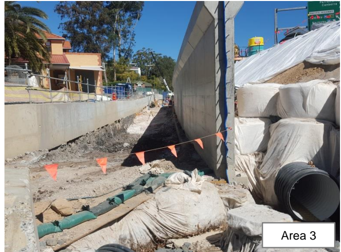
Photo 77: Permanent channel works, including regrading and construction of a low flow channel, geo-fabric and plastic lining, and gabion basalt rock baskets. Photo 78: Outlet of the temporary realignment channel at 2B Burns Road. The section had to be piped due to the construction of a piling pad
