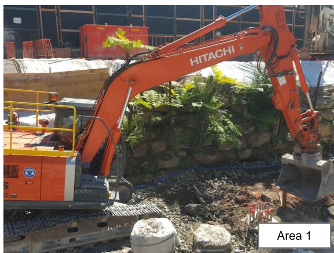
Photo 69: Excavation behind the piles for retaining wall 2, in preparation for the temporary realignment of Cockle Creek. Note the temporary diversion in place directing the clean water flows of Cockle Creek around the work area. Photo 70: Extension of the 1800 pipe outlet at the portal, and the bulka bags acting as the protective barrier for the creek
