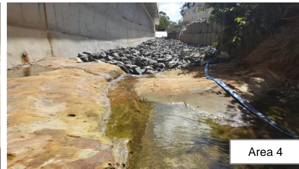
Photo 88 and 89: Sections of Cockle Creek realigned into the permanent channel, with both natural bedrock and basalt rock
