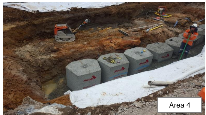
Photo 45: Excavation of the creek bed, for the installation of the mass block wall, noting a temporary creek diversion is in place to divert water around the work area. Photo 46: Commencement of installation of mass blocks
