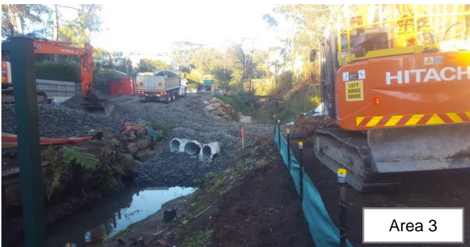
Photo 15: Steel plates removed over the crossing whilst plant travel across the crossing. Photo 16: ERSED controls set up around temporary crossing including a sediment fence, stabilised access on either side of the crossing and sandbag bunding
