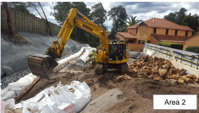
Photo 28: The existing creek bed is being backfilled in preparation for the installation of the plywood fencing. Photo 29: Installation of the plywood fencing.
