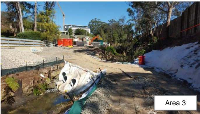
Photo 17: Temporary crossing installation. Photo 18: Installation of temporary crossing at Lochville Street, to attain access on the western side of Cockle Creek
