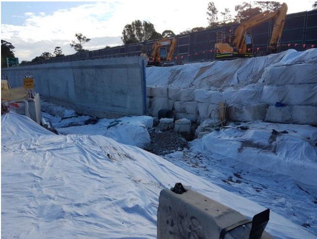
Photo 100 and 101: Area at 2B Burns Road stabilised and secured with geo-fabric, and the excavated channel lined with geo-fabric
