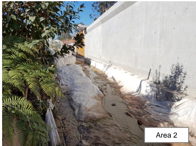
Photo 73 & 74: Temporary realignment of Cockle Creek behind retaining wall 02, with geo-fabric and clean basalt rock lining. Note the pipe is set up but not in use for a temporary diversion
