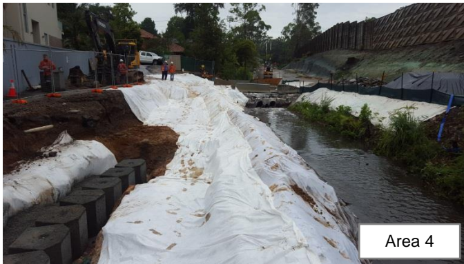
Photo 47: Area 4 during a rain event, with the site team installing heavy duty geo-fabric along the creek bank and around the mass block wall area. Photo 48: Section of mass block wall completed, with geo-fabric lined batter and installation of clean basalt rock in the creek channel
