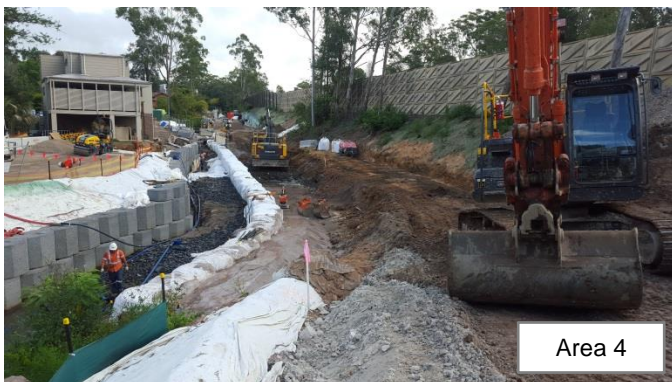
Photo 51 & 52: Continued installation of the bulka bags and plywood fencing, in preparation for the piling pad and piling works
