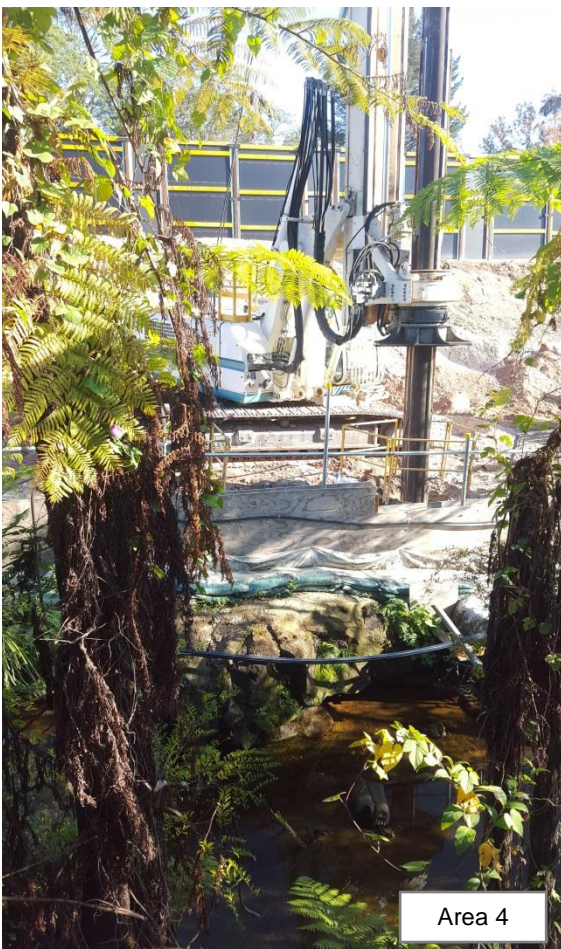
Photo 40: Piling along Cockle Creek
