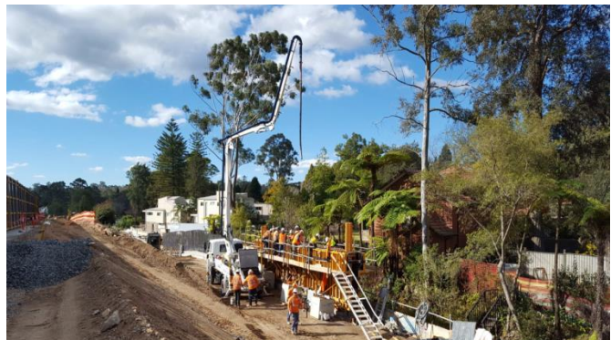
Photo 59 and 60: Concrete pour with a concrete pump into various sections of retaining wall 2
