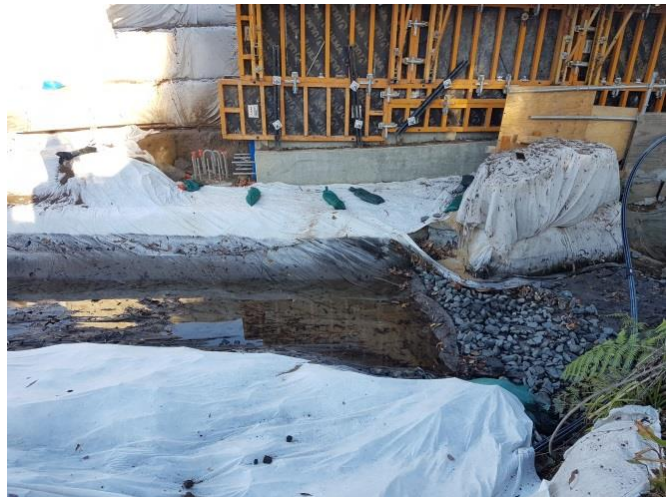
Photo 100 and 101: Area at 2B Burns Road stabilised and secured with geo-fabric, and the excavated channel lined with geo-fabric
