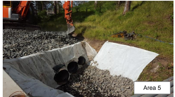
Photo 17: Temporary crossing installation. Photo 18: Installation of temporary crossing at Lochville Street, to attain access on the western side of Cockle Creek
