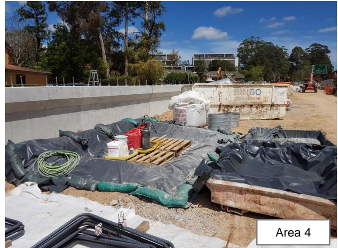
Photo 63: Temporary diversion set up directing the clean water flows of Cockle Creek around the area to be poured. Plastic lining is placed over the creek to ensure any spills or overpours are captured. Photo 64: Concrete washout and chemical bunding in preparation for a concrete pour
