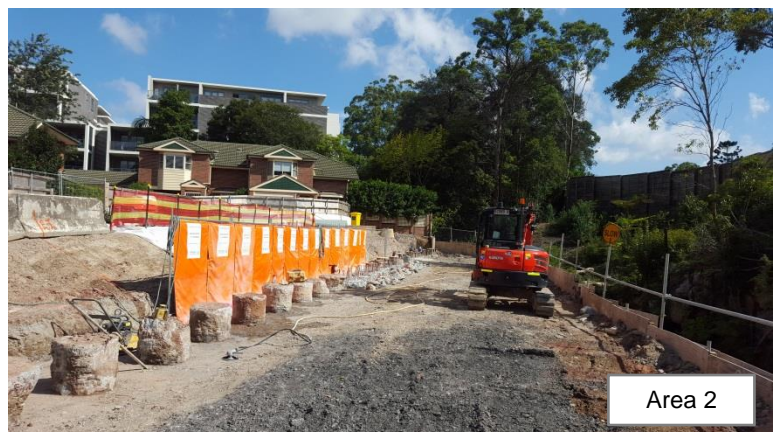
Photo 42: Pile trimming near Cockle Creek, with noise blankets set up
