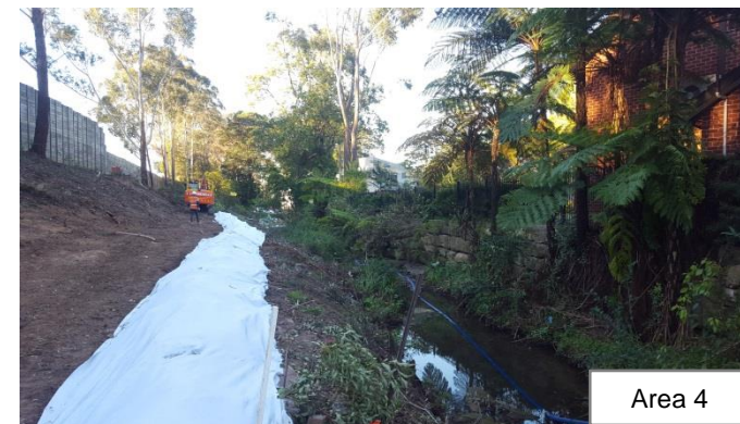
Photo 9 & 10: Clearing progressing on the western side of Cockle Creek, with ERSED controls being progressively installed
