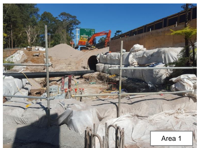
Photo 69: Excavation behind the piles for retaining wall 2, in preparation for the temporary realignment of Cockle Creek. Note the temporary diversion in place directing the clean water flows of Cockle Creek around the work area. Photo 70: Extension of the 1800 pipe outlet at the portal, and the bulka bags acting as the protective barrier for the creek
