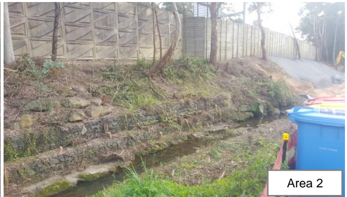
Photo 5 & 6: Area cleared, with the tree stumps and root zone remaining in place on the batters. Note the proximity of the noise wall of the M1 Motorway adjacent to the creek
