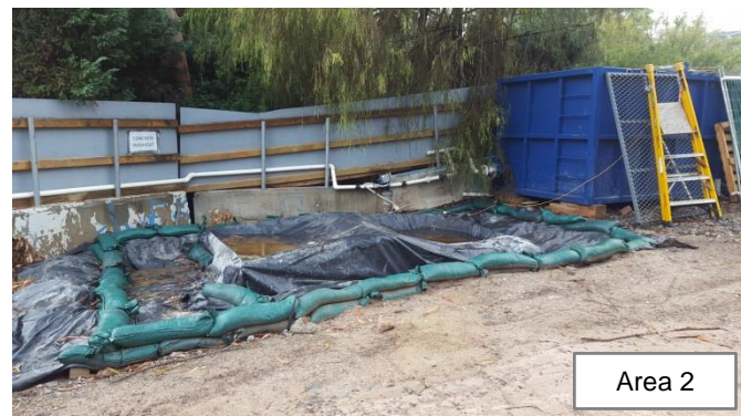
Photo 61 and 62: Concrete delivery and washout set up along Cockle Creek for the retaining wall pours
