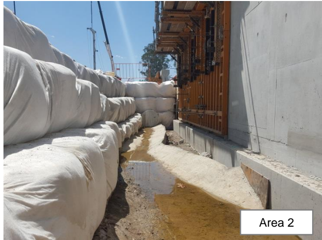
Photo 71: Temporary realignment of Cockle Creek around the piling works at the M120 portal. Photo 72: Temporary realignment of Cockle Creek behind the retaining wall, with the surface water channel being concreted and the low flow channel in place
