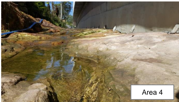
Photo 88 and 89: Sections of Cockle Creek realigned into the permanent channel, with both natural bedrock and basalt rock
