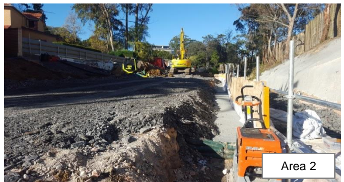
Photo 36: Shotcreted batter along the temporary creek alignment. Photo 37: Concrete poured behind the plywood fencing, with sandbag breaks installed along the alignment to capture any runoff from the piling pad
