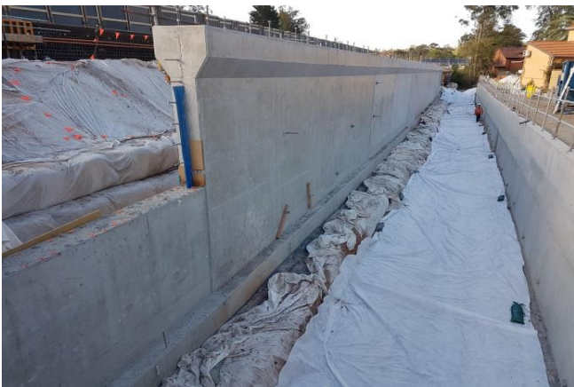
Photo 102: Permanent alignment channel secured with geo-fabric prior to a rain event. Photo 103: Permanent alignment channel following a rain event
