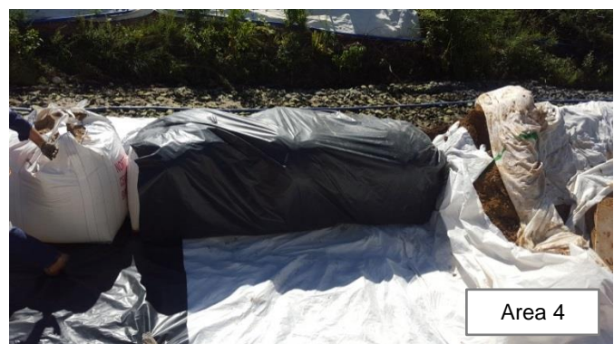
Photo 22 and 23: Temporary creek diversion is in place, whilst the creek bed has been excavated and the bulka bags are being installed, firstly wrapped in plastic and secondly with heavy duty geo-fabric. Note a small section of the creek bed has been excavated to ensure the construction activity is complete at the end of the shift, and to return natural the creek flows with no disturbance
