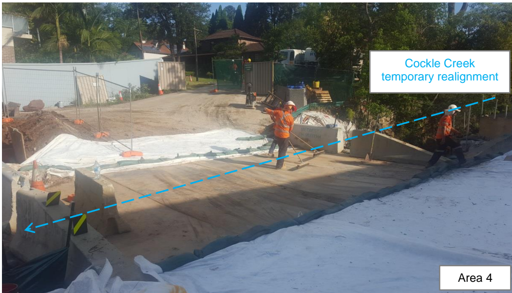
Photo 20: Temporary crossing at Bareena Avenue
