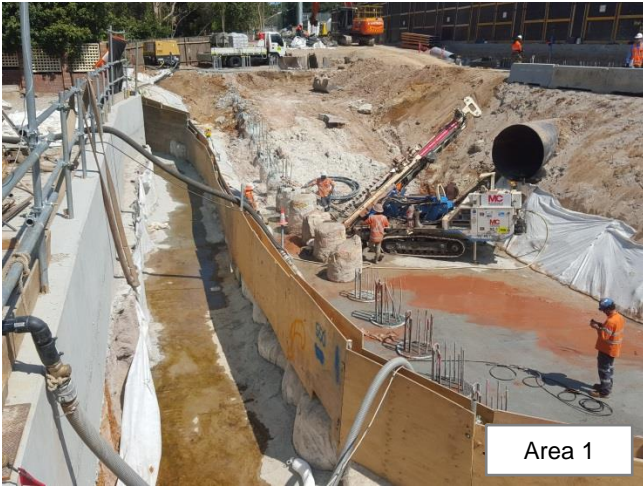
Photo 71: Temporary realignment of Cockle Creek around the piling works at the M120 portal. Photo 72: Temporary realignment of Cockle Creek behind the retaining wall, with the surface water channel being concreted and the low flow channel in place
