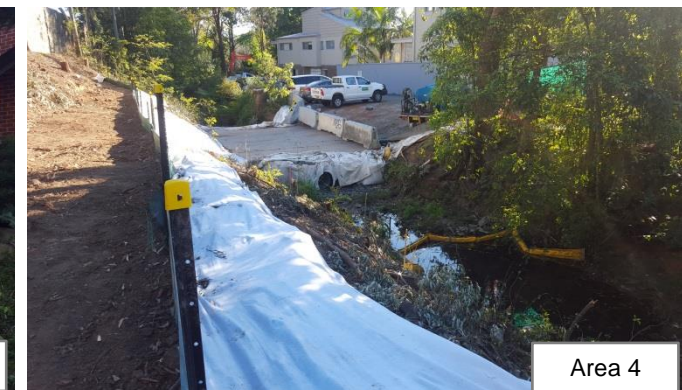
Photo 9 & 10: Clearing progressing on the western side of Cockle Creek, with ERSED controls being progressively installed
