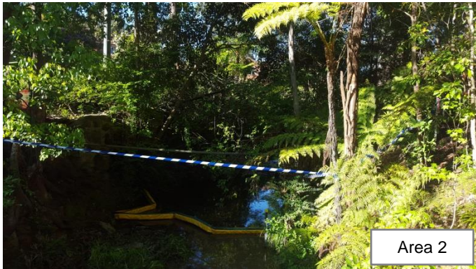
Photo 3 & 4: Clearing tape and sensitive area fencing delineating the vegetation area to be cleared, and the boom installed as secondary protection in the event of an environmental spill or additional debris
