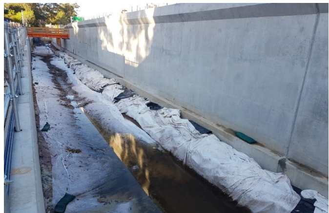
Photo 102: Permanent alignment channel secured with geo-fabric prior to a rain event. Photo 103: Permanent alignment channel following a rain event
