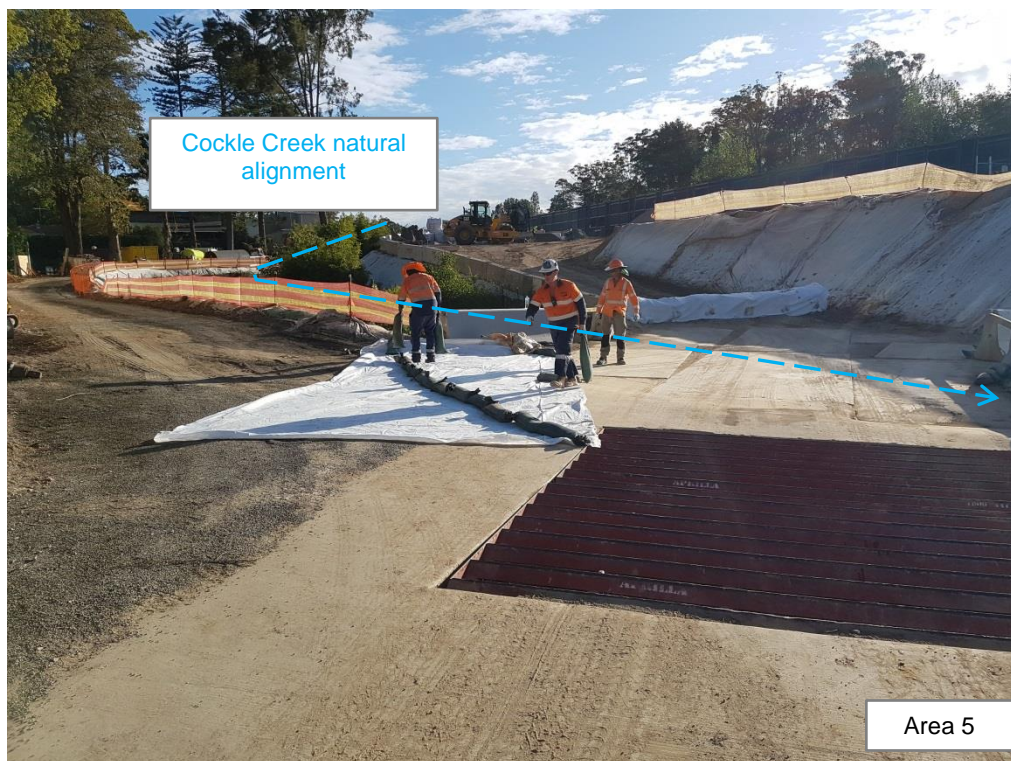
Photo 21: Temporary crossing at Lochville Street
