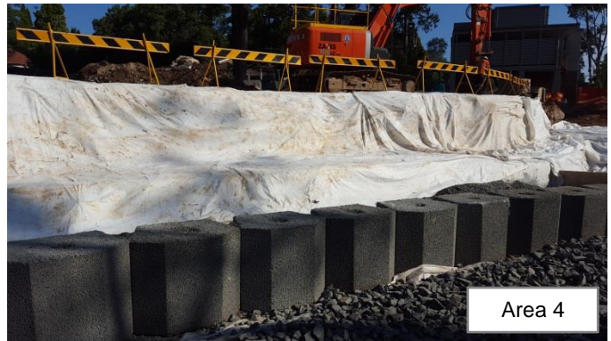
Photo 47: Area 4 during a rain event, with the site team installing heavy duty geo-fabric along the creek bank and around the mass block wall area. Photo 48: Section of mass block wall completed, with geo-fabric lined batter and installation of clean basalt rock in the creek channel
