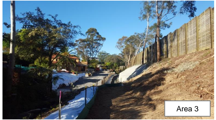
Photo 32: Completed plywood fencing and backfill for the piling pad, noting the sandbag breaks in place along the alignment to prevent potential erosion. Photo 33: View from 2B Burns Road looking southwards towards the completed temporary creek realignment
