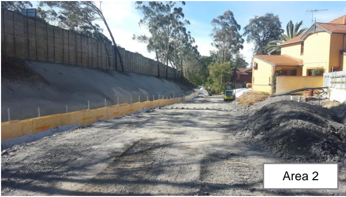
Photo 32: Completed plywood fencing and backfill for the piling pad, noting the sandbag breaks in place along the alignment to prevent potential erosion. Photo 33: View from 2B Burns Road looking southwards towards the completed temporary creek realignment
