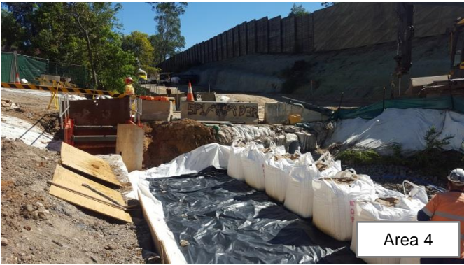
Photo 24 and 25: Small section of the creek bed at Bareena Avenue, with the bulka bags being installed progressively
