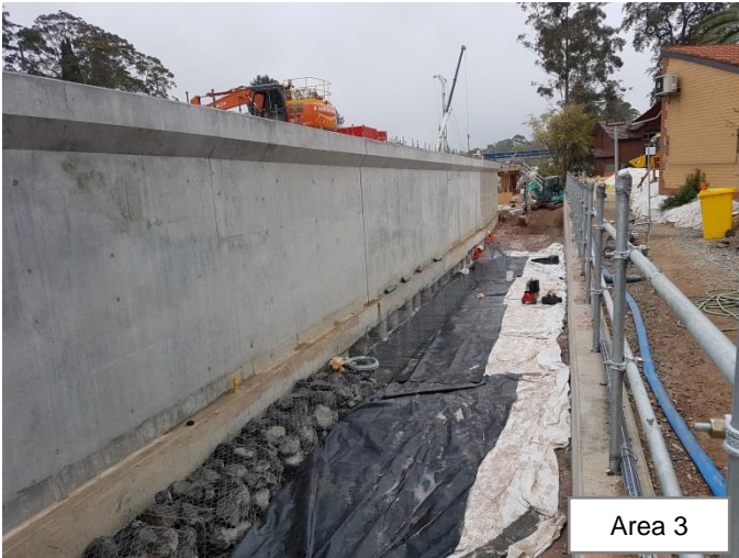
Photo 77: Permanent channel works, including regrading and construction of a low flow channel, geo-fabric and plastic lining, and gabion basalt rock baskets. Photo 78: Outlet of the temporary realignment channel at 2B Burns Road. The section had to be piped due to the construction of a piling pad
