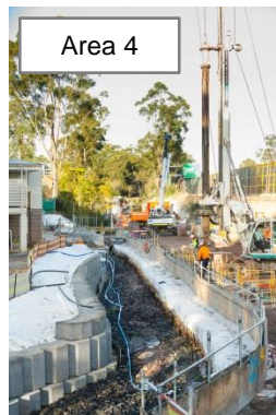
Photo 53: Extension of mass block wall, and piling pad preparation. Photo 54: Piling commencement following the installation of bulka bags and plywood fencing. Photo 55: Concrete management during the installation of the plywood fencing and mass block wall
