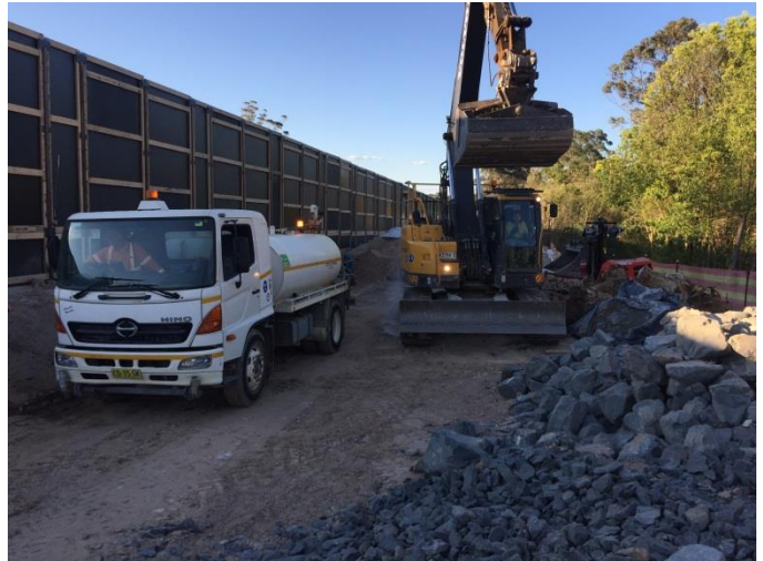
Photo 77: Permanent channel works, including regrading and construction of a low flow channel, geo-fabric and plastic lining, and gabion basalt rock baskets. Photo 78: Outlet of the temporary realignment channel at 2B Burns Road. The section had to be piped due to the construction of a piling pad
