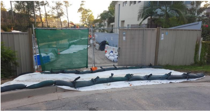
Photo 96 & 97: Shutdown controls at the access points to site.
