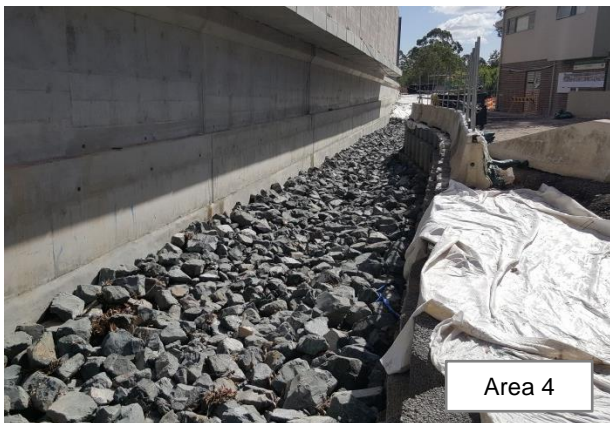
Photo 86 and 87: Sections of Cockle Creek realigned into the permanent channel, with both natural bedrock and basalt rock
