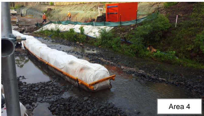
Photo 49: Commencement of installation of bulka bag wall for the creek realignment, following a rain event. Photo 50: Installation of bulka bag and plywood fencing along area 4, during a temporary creek diversion around the works (the 3 pipes along the rock)
