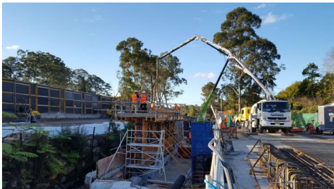
Photo 59 and 60: Concrete pour with a concrete pump into various sections of retaining wall 2
