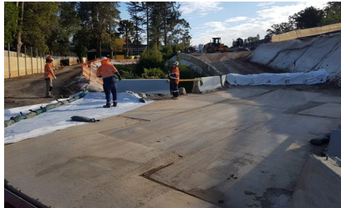
Photo 92 and 93: Progressively installing bulka bags wrapped and secured with geo-fabric at Lochville Street temporary crossing, prior to a rain event
