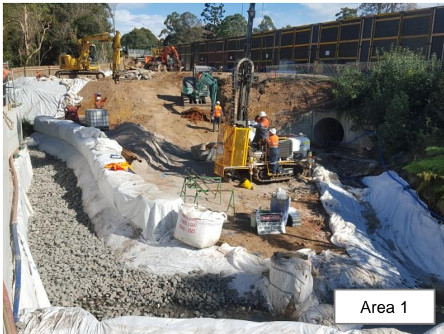
Photo 65: Cockle creek temporarily realigned around the piling and soil anchor works. Photo 66: Cockle Creek following a rain event
