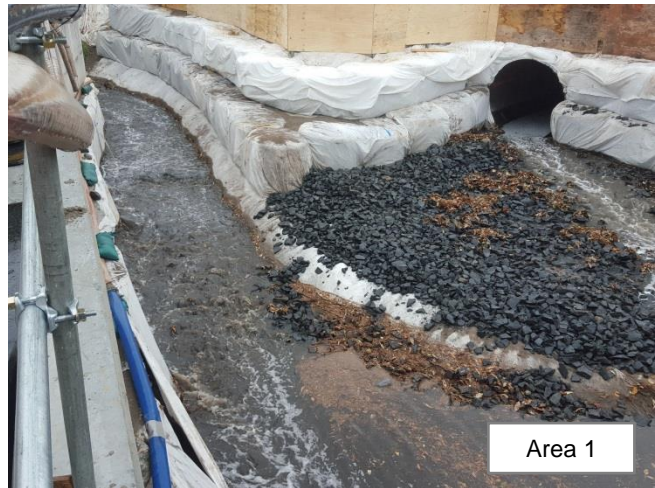
Photo 65: Cockle creek temporarily realigned around the piling and soil anchor works. Photo 66: Cockle Creek following a rain event
