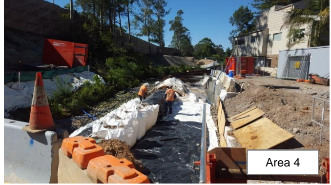
Photo 24 and 25: Small section of the creek bed at Bareena Avenue, with the bulka bags being installed progressively
