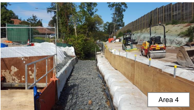
Photo 38: Section at Bareena Avenue realigned with bulka bag and plywood fencing installed. Photo 39: Temporary crossing at 2B Burns Road
