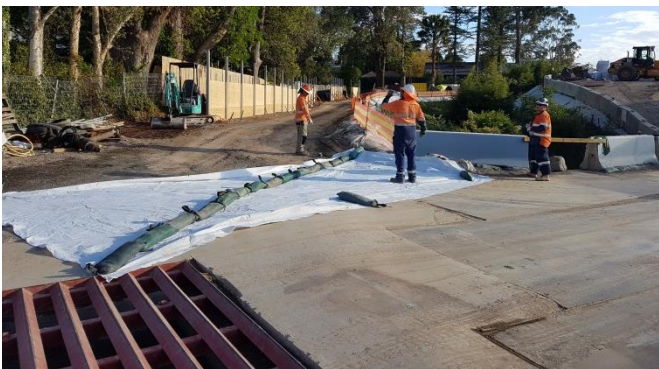
Photo 94: Sandbag bund directing any dirty water runoff from the access track to the rumble grid, which was specifically designed to have the capacity of a small sump due to the access location being next to the creek. Photo 95: Post rain showing the sediment captured with the bunding, preventing any dirty water runoff into Cockle Creek
