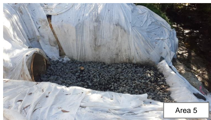
Photo 58: Additional geo-fabric and basalt rock placed in preparation for the connection
