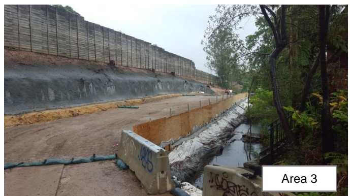
Photo 38: Section at Bareena Avenue realigned with bulka bag and plywood fencing installed. Photo 39: Temporary crossing at 2B Burns Road
