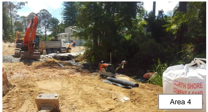
Photo 34 and 35: Installation of bulka bags in section of the creek between 2B Burns Road and Bareena Avenue, where the natural creek bed is unstable. Plywood fencing with concrete was installed as a protective measure for the creek, in preparation for the piling activity
