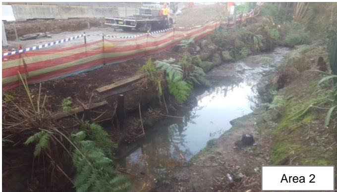
Photo 5 & 6: Area cleared, with the tree stumps and root zone remaining in place on the batters. Note the proximity of the noise wall of the M1 Motorway adjacent to the creek
