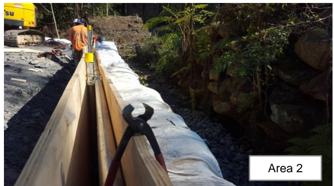
Photo 28: The existing creek bed is being backfilled in preparation for the installation of the plywood fencing. Photo 29: Installation of the plywood fencing.
