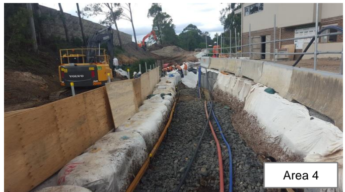
Photo 49: Commencement of installation of bulka bag wall for the creek realignment, following a rain event. Photo 50: Installation of bulka bag and plywood fencing along area 4, during a temporary creek diversion around the works (the 3 pipes along the rock)
