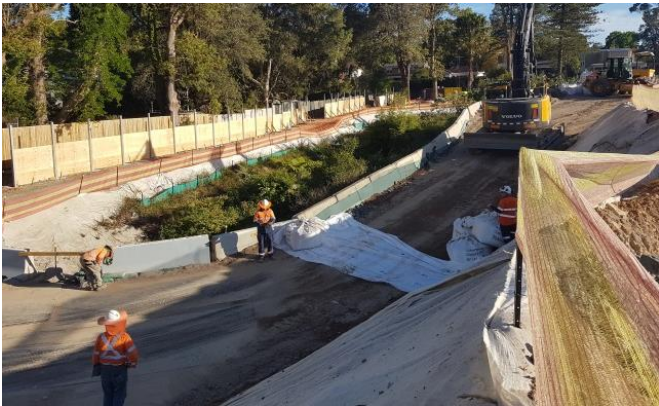
Photo 92 and 93: Progressively installing bulka bags wrapped and secured with geo-fabric at Lochville Street temporary crossing, prior to a rain event
