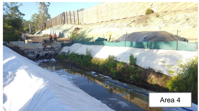
Photo 43: Clearing of tree stumps within the creek bed for the mass block wall installation. Photo 44: Heavy duty geo-fabric used as a temporary measure to stabilise the cleared creek banks, prior to the installation of the bulka bag and plywood fencing
