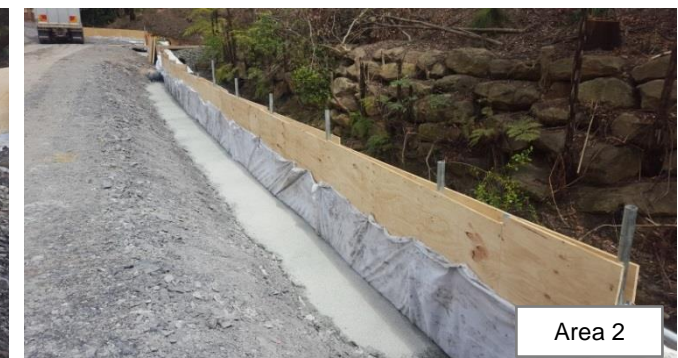
Photo 30 and 31: Completed plywood fencing with concrete backfill along the creek realignment, in preparation for the piling pad
