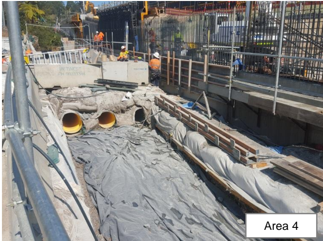
Photo 63: Temporary diversion set up directing the clean water flows of Cockle Creek around the area to be poured. Plastic lining is placed over the creek to ensure any spills or overpours are captured. Photo 64: Concrete washout and chemical bunding in preparation for a concrete pour
