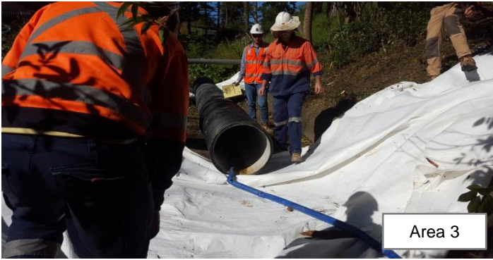
Photo 13: Temporary creek diversion in place whilst clearing the creek bed, placing geo-fabric, clean rock and pipes. Photo 14: Clean basalt rock placed on top of the temporary crossing and an additional layer of geo-fabric to secure the rock
