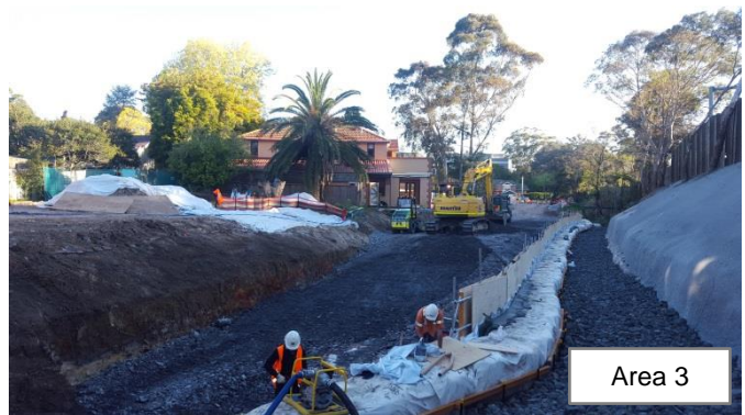
Photo 26: Section of the creek bed at Burns Road looking towards 2B Burns Road (north), where the creek bed has been excavated and bulka bags have been installed. A temporary creek diversion is in place (see the blue pipe), due to the excavation works being in close proximity. The batter has been shotcreted to limit the disturbance to the western side of the creek, and reduce maintenance (refixing/replacing geo-fabric).
