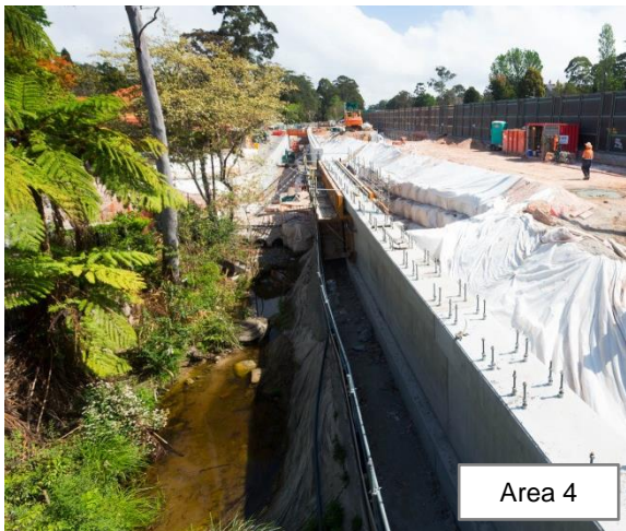
Photo 81 and 82: Batters from the piling pad covered in geo-fabric
