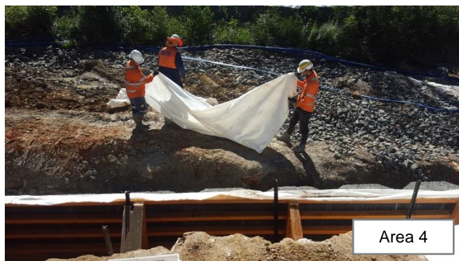
Photo 22 and 23: Temporary creek diversion is in place, whilst the creek bed has been excavated and the bulka bags are being installed, firstly wrapped in plastic and secondly with heavy duty geo-fabric. Note a small section of the creek bed has been excavated to ensure the construction activity is complete at the end of the shift, and to return natural the creek flows with no disturbance
