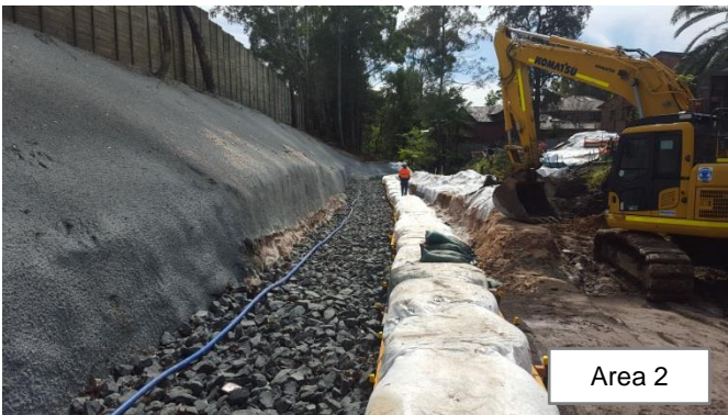
Photo 26: Section of the creek bed at Burns Road looking towards 2B Burns Road (north), where the creek bed has been excavated and bulka bags have been installed. A temporary creek diversion is in place (see the blue pipe), due to the excavation works being in close proximity. The batter has been shotcreted to limit the disturbance to the western side of the creek, and reduce maintenance (refixing/replacing geo-fabric).
