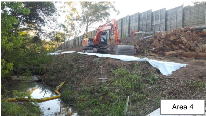
Photo 7: Commencement of installation of geo-fabric bunded batter along the western side of Cockle Creek, with marine boom installed as a precaution measure. Photo 8: Temporary crossing at Barena Avenue installed, with completed geo-fabric bund and sedimentation fence
