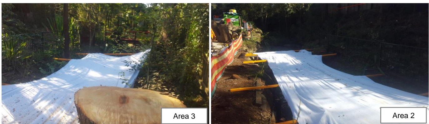
Photo 1 & 2: Timber frame with geo-fabric, to capture any debris during clearing activity
