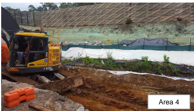
Photo 45: Excavation of the creek bed, for the installation of the mass block wall, noting a temporary creek diversion is in place to divert water around the work area. Photo 46: Commencement of installation of mass blocks
