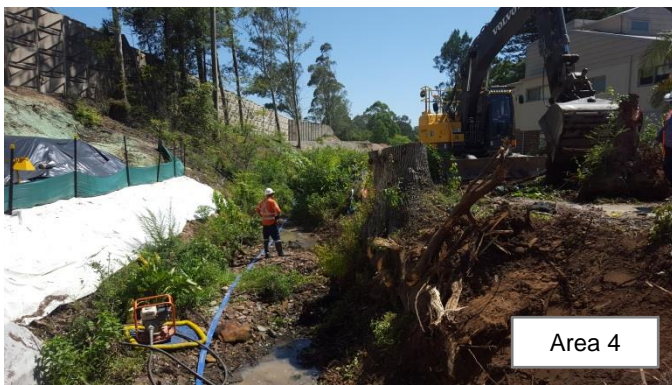
Photo 43: Clearing of tree stumps within the creek bed for the mass block wall installation. Photo 44: Heavy duty geo-fabric used as a temporary measure to stabilise the cleared creek banks, prior to the installation of the bulka bag and plywood fencing
