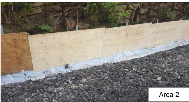
Photo 30 and 31: Completed plywood fencing with concrete backfill along the creek realignment, in preparation for the piling pad
