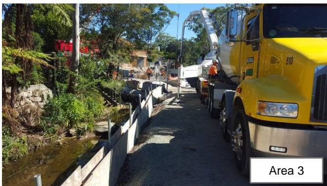
Photo 61 and 62: Concrete delivery and washout set up along Cockle Creek for the retaining wall pours
