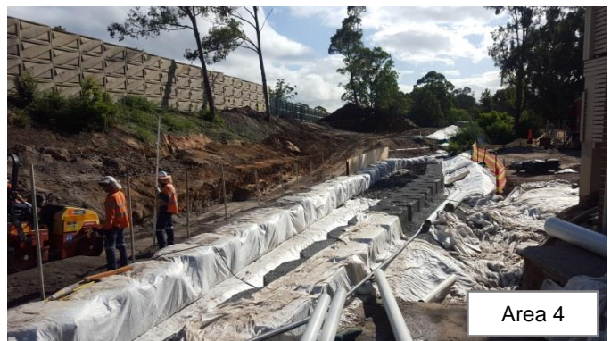
Photo 51 & 52: Continued installation of the bulka bags and plywood fencing, in preparation for the piling pad and piling works
