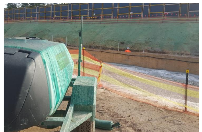
Photo 98: Area stabilised with soil binder and batters secured with geo-fabric along Cockle Creek. Photo 99: Soil binder unit utilising Vital Chemical soil binder products, and sprayed batter in the background
