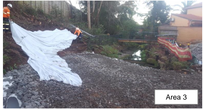
Photo 13: Temporary creek diversion in place whilst clearing the creek bed, placing geo-fabric, clean rock and pipes. Photo 14: Clean basalt rock placed on top of the temporary crossing and an additional layer of geo-fabric to secure the rock
