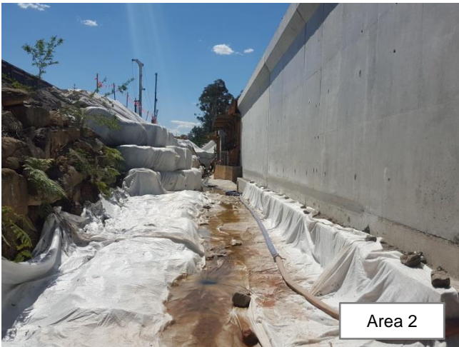
Photo 73 & 74: Temporary realignment of Cockle Creek behind retaining wall 02, with geo-fabric and clean basalt rock lining. Note the pipe is set up but not in use for a temporary diversion
