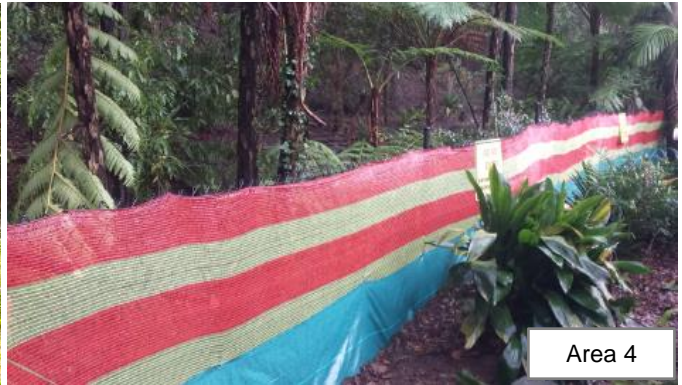
Photo 3 & 4: Clearing tape and sensitive area fencing delineating the vegetation area to be cleared, and the boom installed as secondary protection in the event of an environmental spill or additional debris
