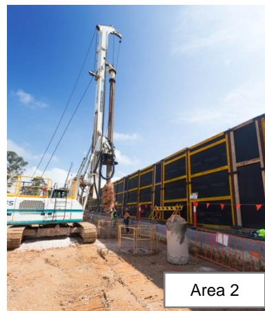
Photo 83: Bailey Bridge with environmental controls installed at Burns Road. Photo 84: Piling the remaining retaining wall adjacent to the M1 Pacific Motorway. Photo 85: Batters along the piling pad sprayed with Vital Chemicals soil binder
