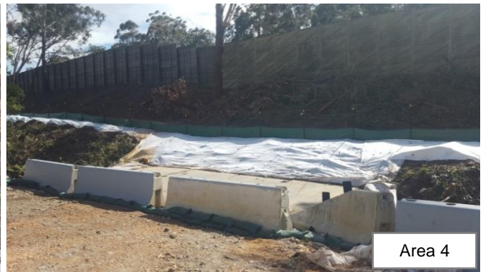
Photo 7: Commencement of installation of geo-fabric bunded batter along the western side of Cockle Creek, with marine boom installed as a precaution measure. Photo 8: Temporary crossing at Barena Avenue installed, with completed geo-fabric bund and sedimentation fence
