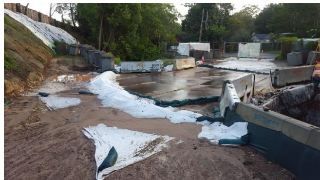
Photo 94: Sandbag bund directing any dirty water runoff from the access track to the rumble grid, which was specifically designed to have the capacity of a small sump due to the access location being next to the creek. Photo 95: Post rain showing the sediment captured with the bunding, preventing any dirty water runoff into Cockle Creek
