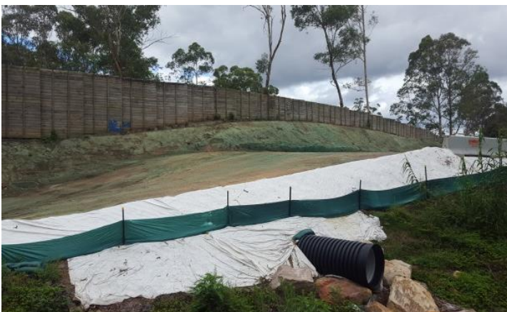
Photo 98: Area stabilised with soil binder and batters secured with geo-fabric along Cockle Creek. Photo 99: Soil binder unit utilising Vital Chemical soil binder products, and sprayed batter in the background
