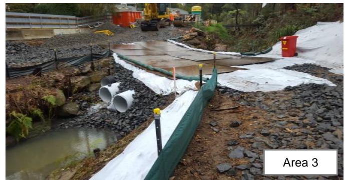
Photo 15: Steel plates removed over the crossing whilst plant travel across the crossing. Photo 16: ERSED controls set up around temporary crossing including a sediment fence, stabilised access on either side of the crossing and sandbag bunding
