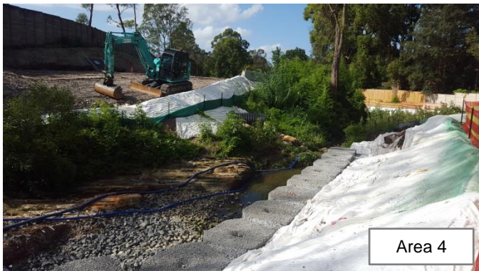
Photo 53: Extension of mass block wall, and piling pad preparation. Photo 54: Piling commencement following the installation of bulka bags and plywood fencing. Photo 55: Concrete management during the installation of the plywood fencing and mass block wall
