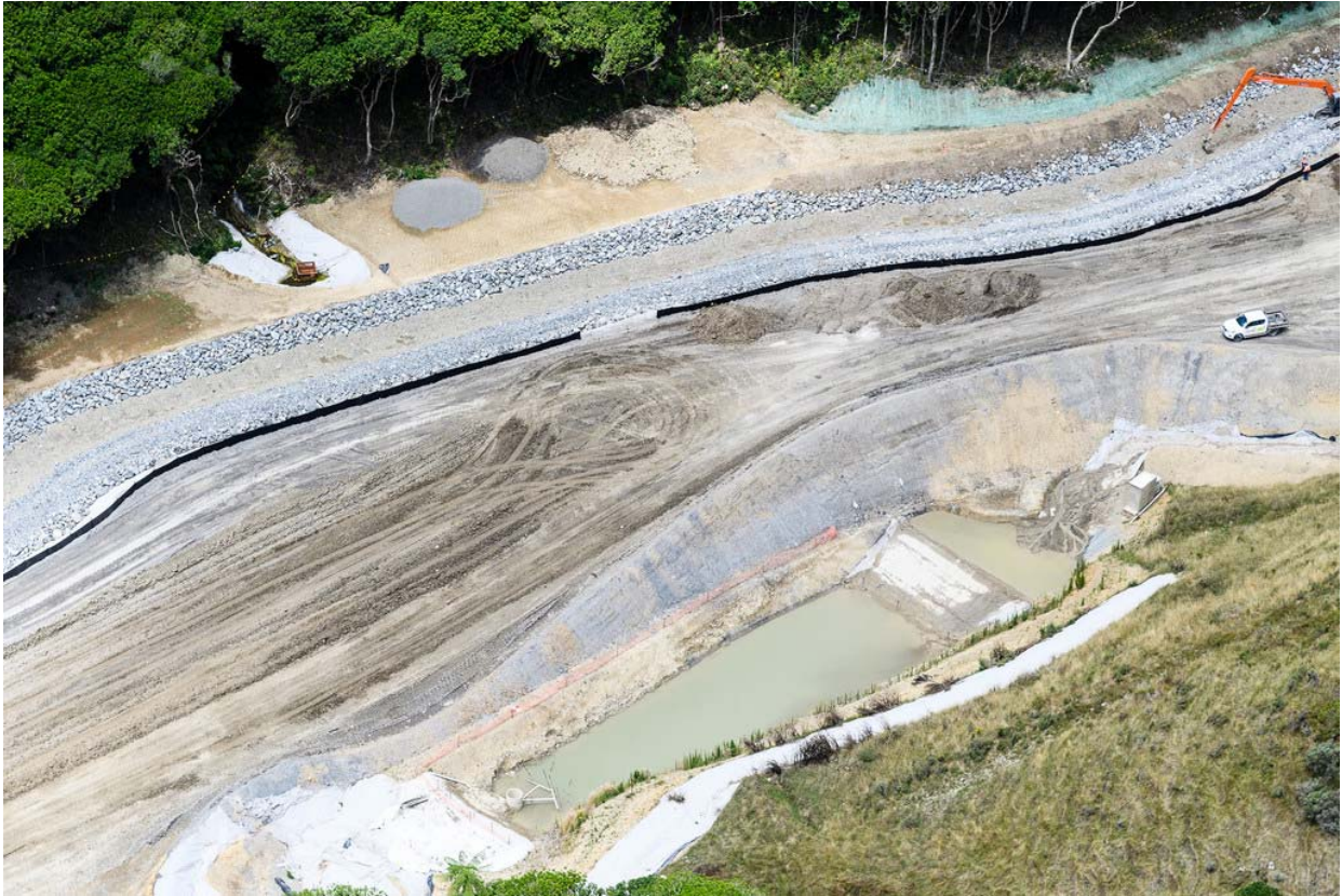
Figure 13: Te Puka diversion under construction
