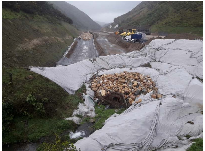
Figure 5: Inlet of temporary stream diversion pipe
