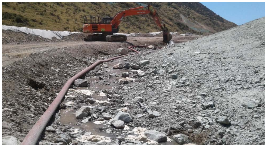
Figure 10: Washing in of stream salvage prior to livening to promote surface flow
