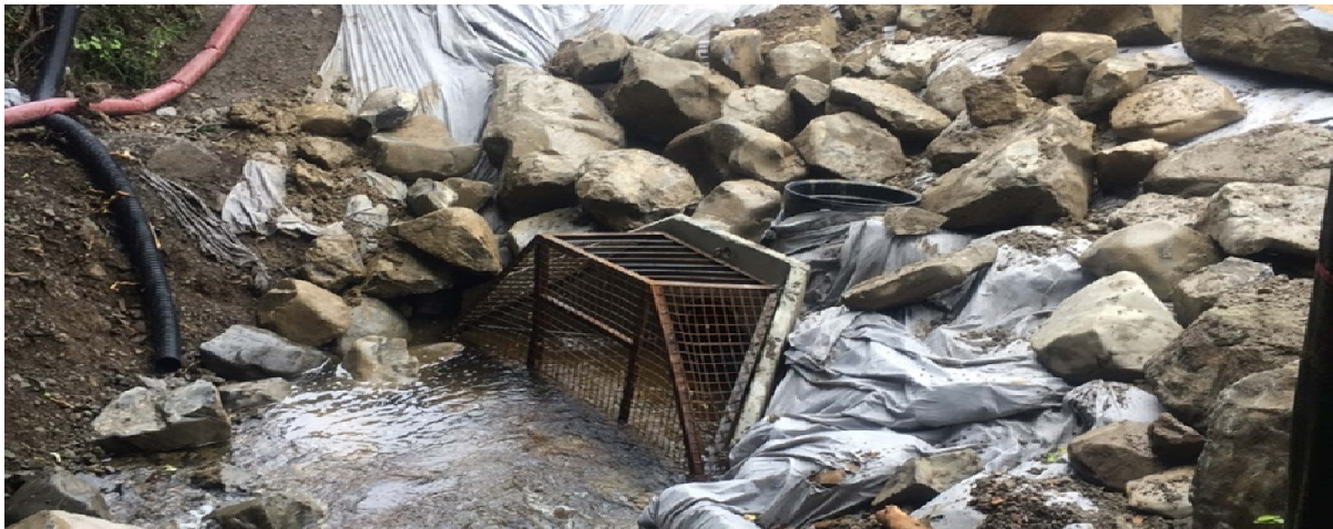
Figure 6: Double inlet structure
