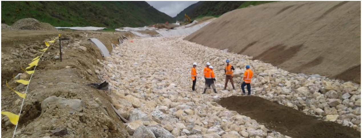
Figure 9: Horokiri permanent diversion
