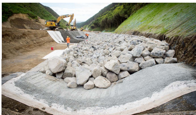
Figure 1: The new permanent Te Puka Stream channel under construction.
