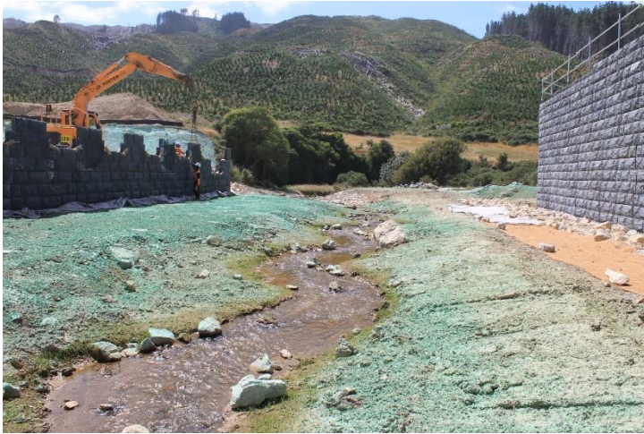
Figure 11. Bridge 6 Stream diversion immediately post livening
