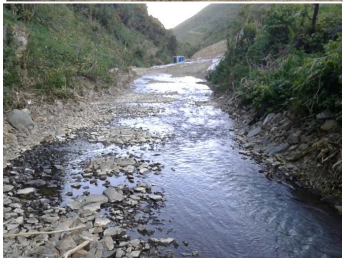
Figure 8: Bedding Rock placed in stream
