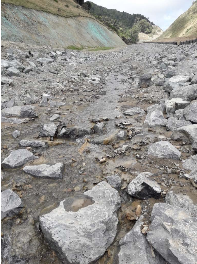
Figure 16: Te Puka Stream diversion post livening
