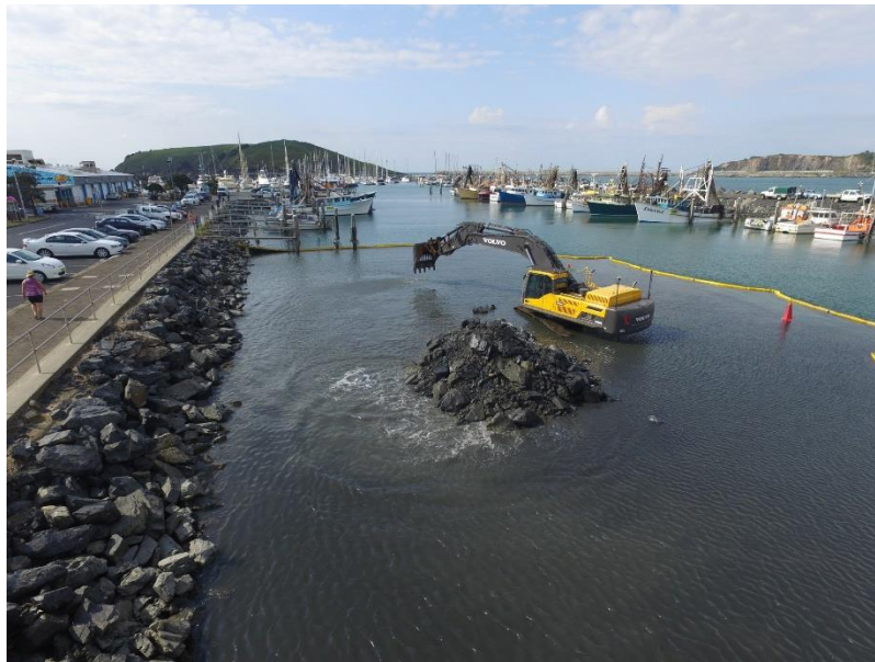
Recovery of submarine section of the slipway.
