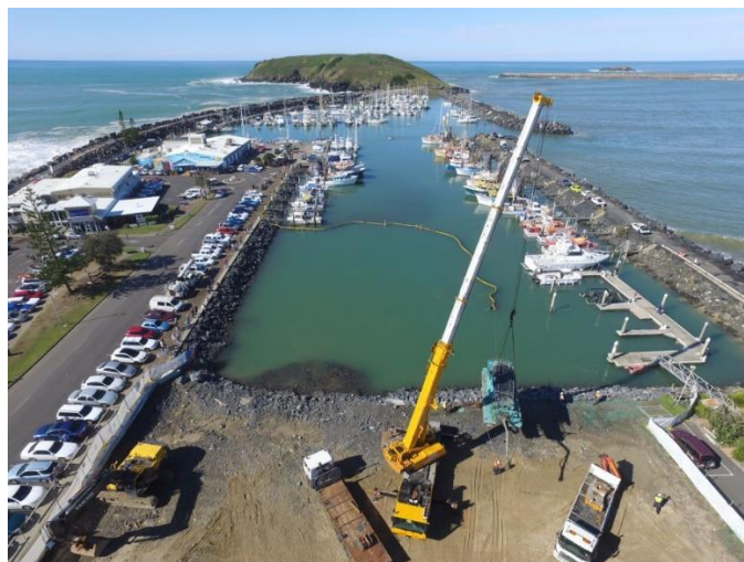
Franna Crane Lifting In Dredge AS THE East coast low subsides
