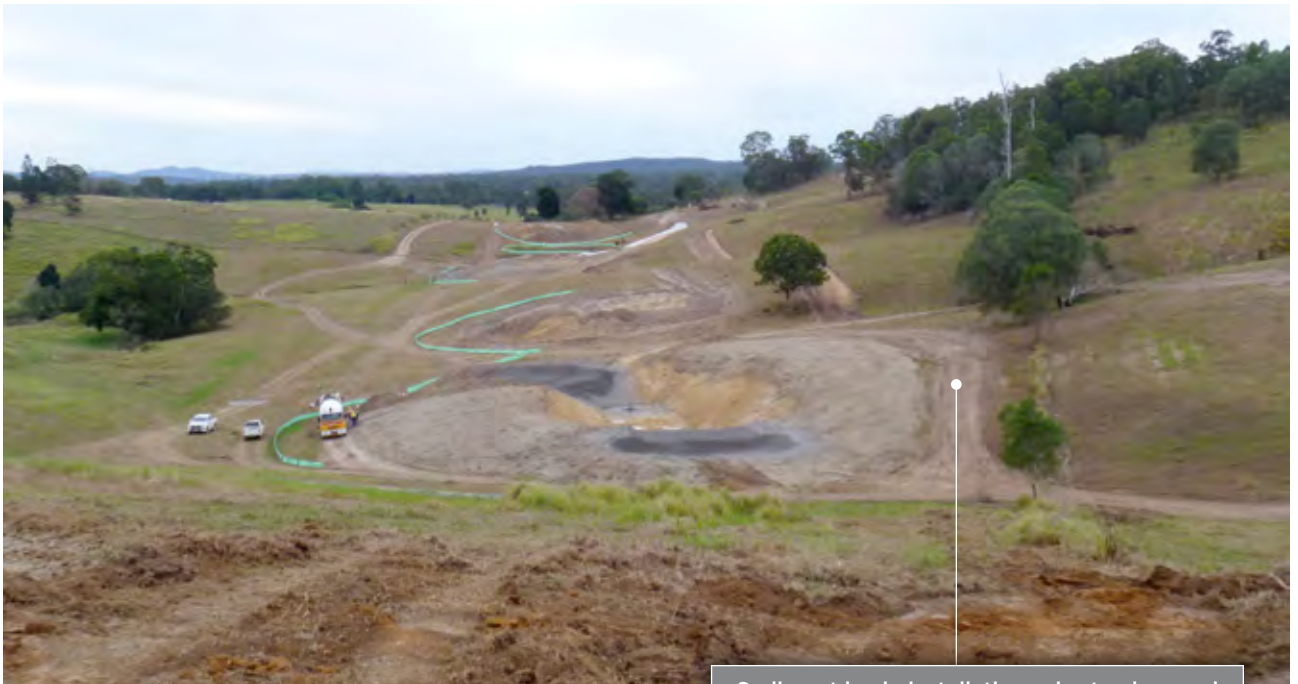
Basin installation amongst heavy vegetation: in-situ mulch used for groundcover and berm at toe of basin until batters were vegetated
