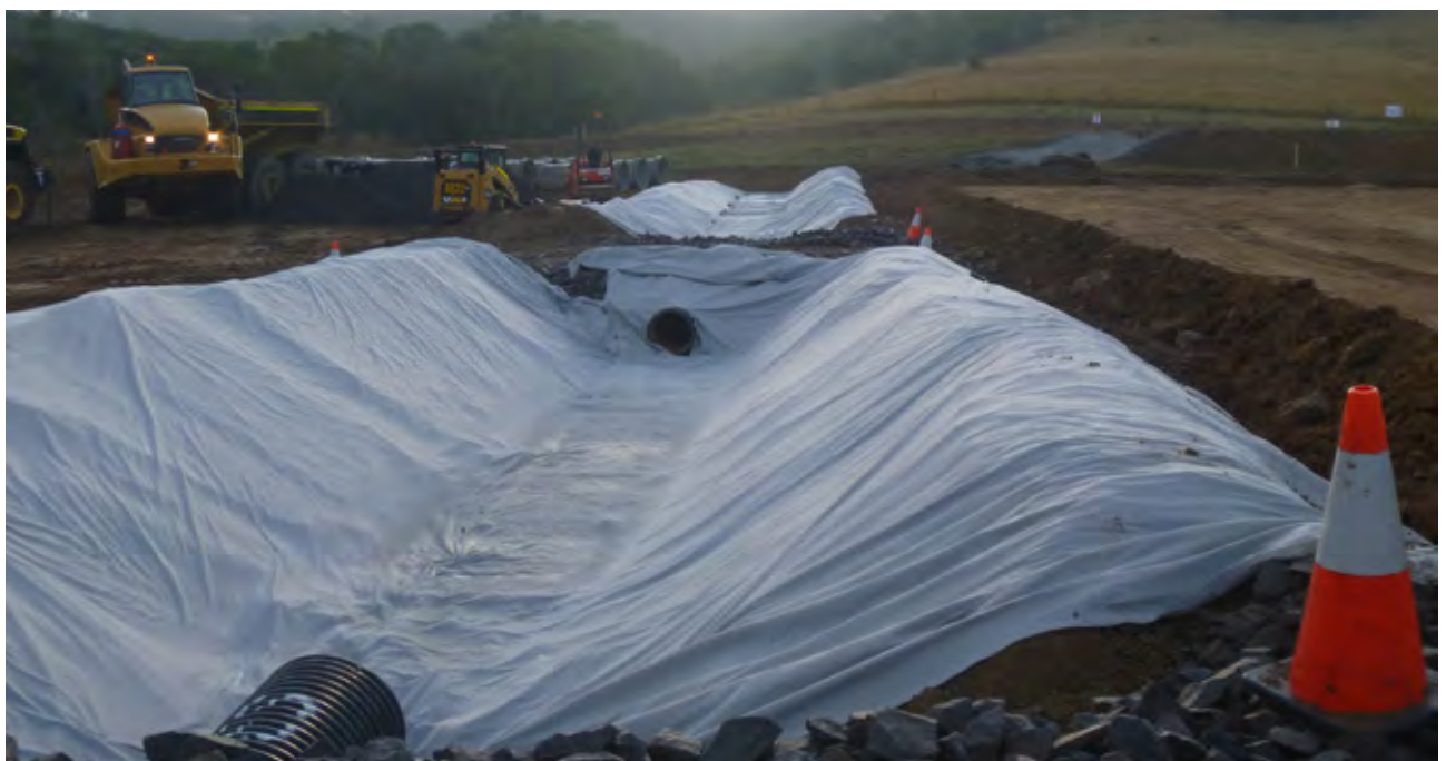
Temporary clean-water cross-drainage
