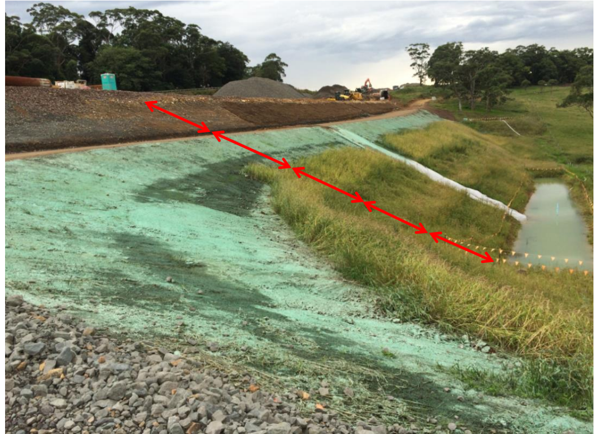
Fill 8 clearly demonstrates each layer of hydromulch in the constructed fill.
