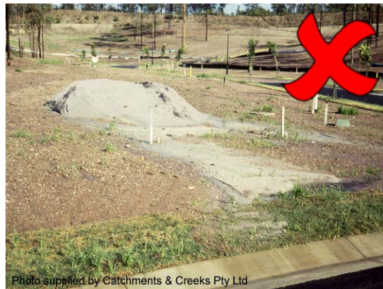
Photo 2 – Sand stockpile inappropriately located within an overland flow path
