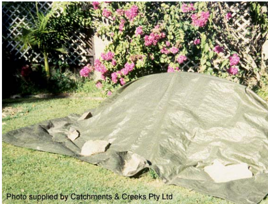
Photo 5 – Stockpile protected with impervious cover
