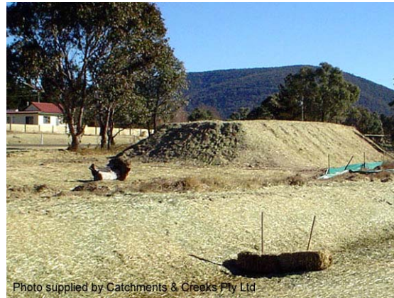
Photo 6 – Earth stockpile protected with mulch
