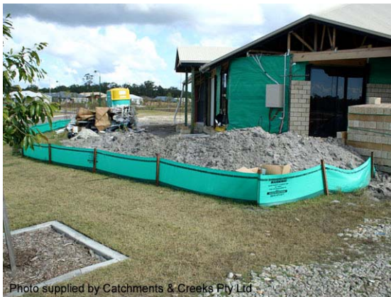
Photo 1 – Soil stockpile located within sediment control envelope
