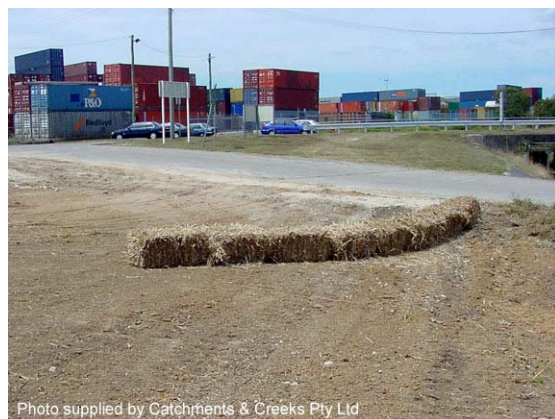
Photo 4 – Straw bales can be used for the temporary diversion of up-slope runoff
