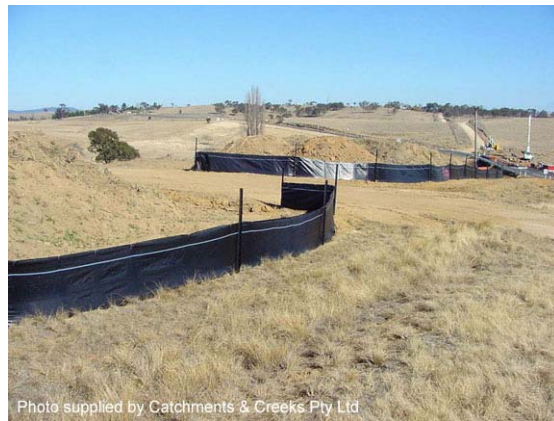
Photo 8 – Sediment fence placed down-slope of soil stockpile
