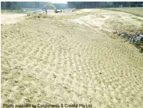
Roughened earth batter
