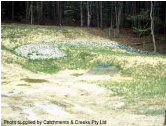
Spillway formed within virgin soil
