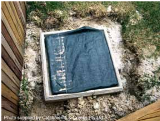
Fabric wrap inlet protection
