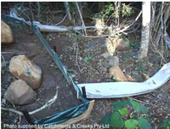
Filter tube dam sediment trap
