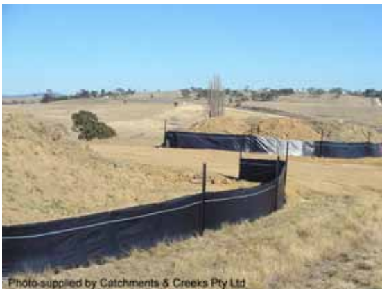
Sediment control down-slope of stockpile
