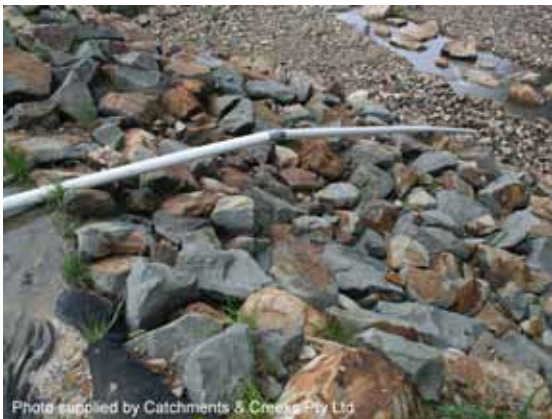
Seepage control a spillway crest
