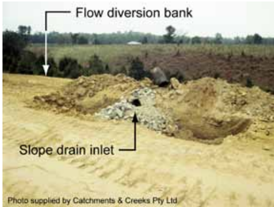
Sediment traps each side of pipe inlet
