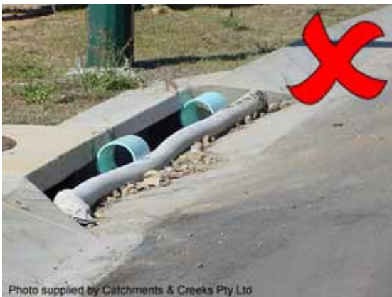
Photo supplied by Catchments & Creeks Pty Ltd Inappropriate on-grade sediment trap
