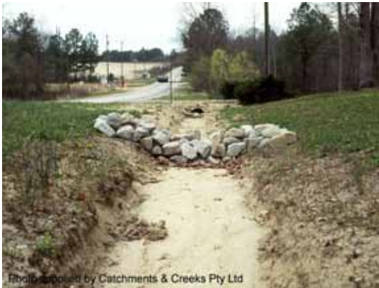
Rock check dam
