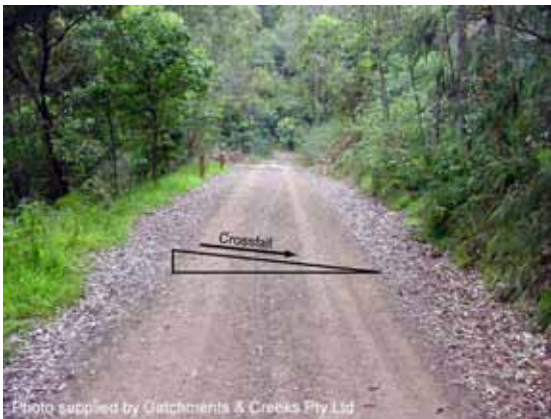
Dirt road with in-fall drainage
