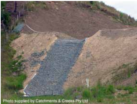
Rock mattress lined spillway chute
