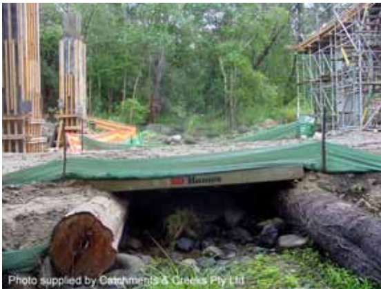
Temporary access construction bridge
