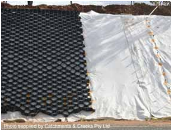
Installation on road batter
