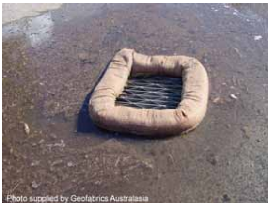
Filter sock drop inlet protection
