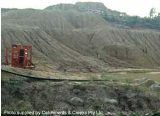
De-watering of basin
