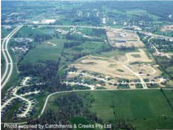
Staged land clearing
