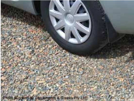
Gravel-stabilised car park
