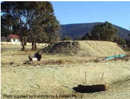
Long-term stockpile covered with mulch
