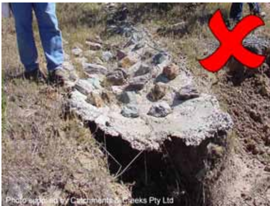
Tunnel erosion
