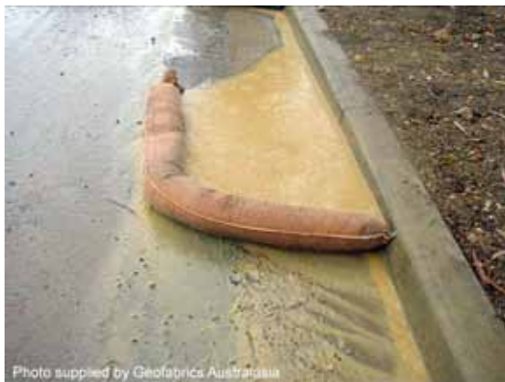
Filter sock sediment trap
