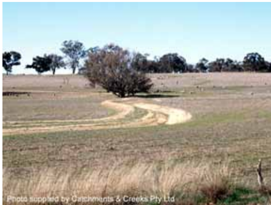
Large catch drain
