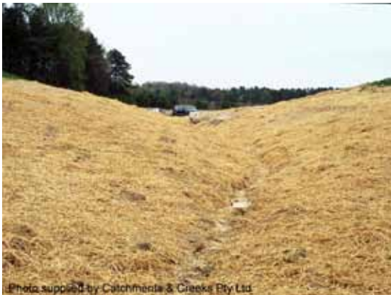
Soil stabilisation with stabilised mulch
