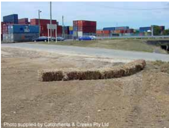
Straw bale flow diversion bank under construction (yet to be staked)
