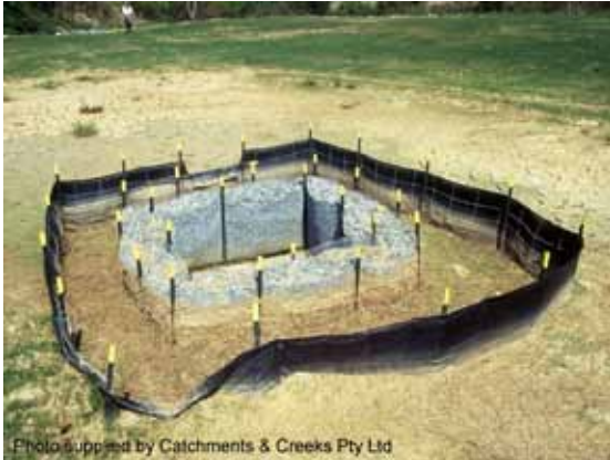
Sediment weir (field inlet protection)
