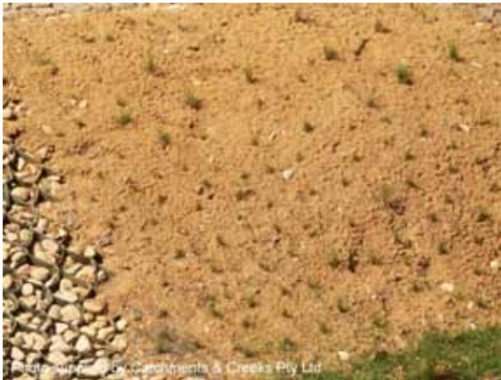
Bonded fibre matrix
