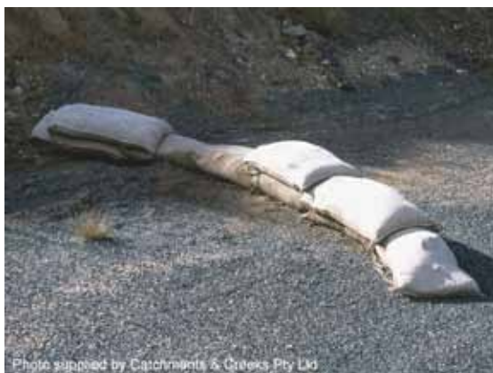
Sandbag sediment trap
