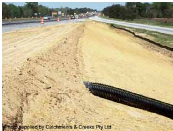
Flow diversion bank controlling flow entry
