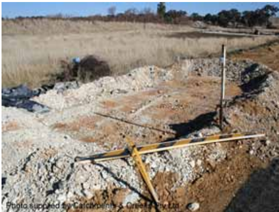
Concrete truck wash-out point
