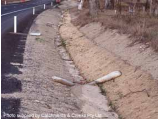
Check dam sediment trap
