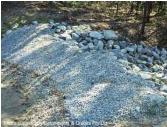
Rock filter dam - aggregate filter
