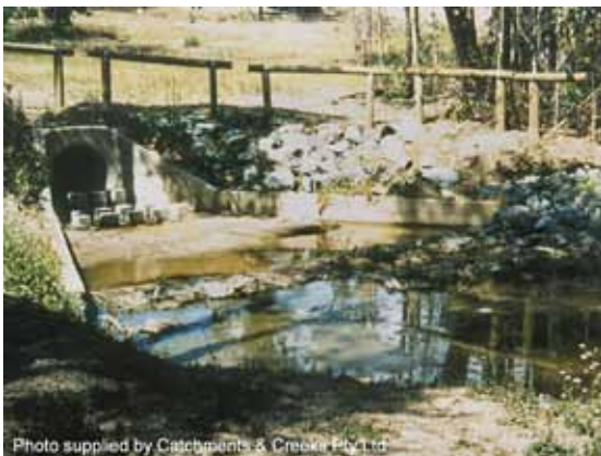
Excavated sediment trap
