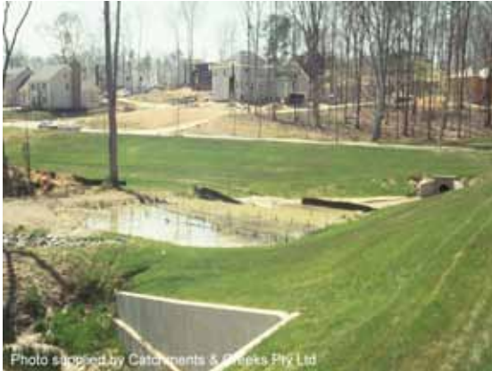
Coarse sediment trap
