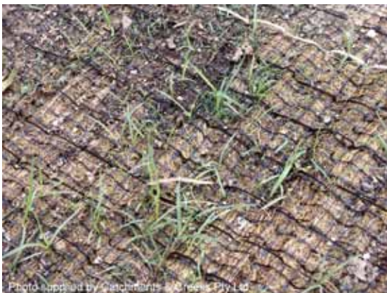
Turf reinforcement mat
