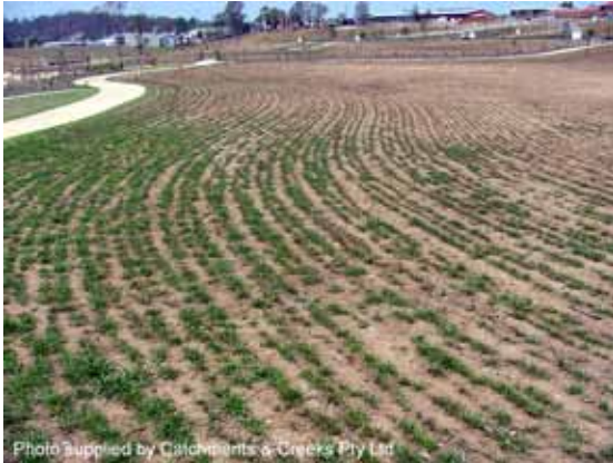
Application of a temporary grasses
