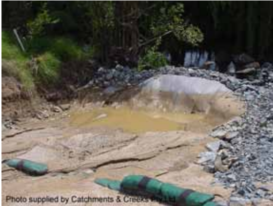
Rock filter dam - geotextile filter
