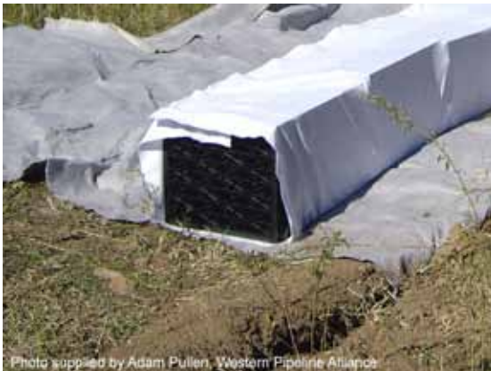
Modular sediment trap being installed
