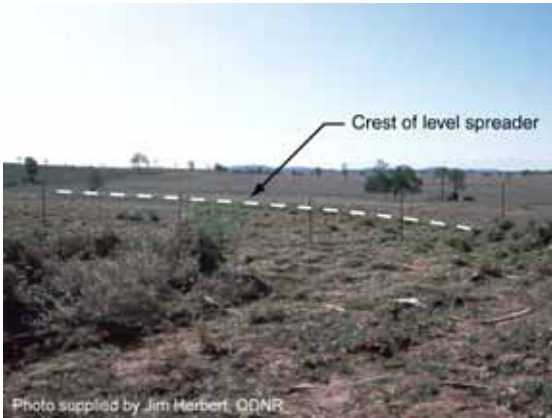
Level spreader used to release road runoff into the adjacent farmland
