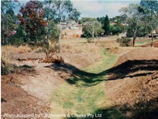
Turf lined diversion drain
