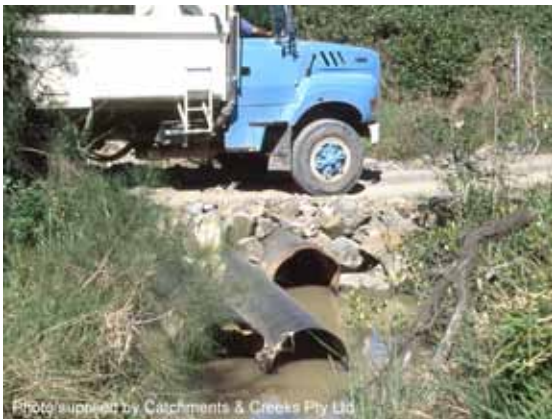
Temporary pipe culvert
