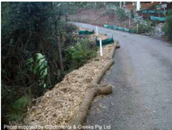
Fibre roll sediment trap
