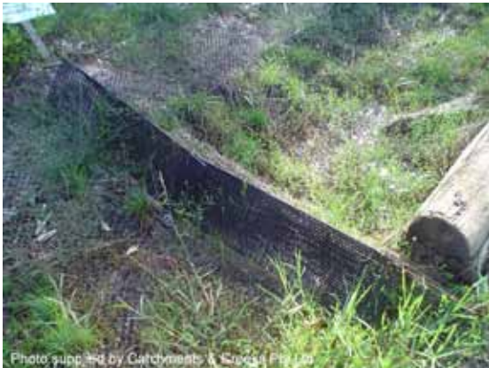
Triangular ditch check
