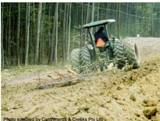
Scarifying the soil surface
