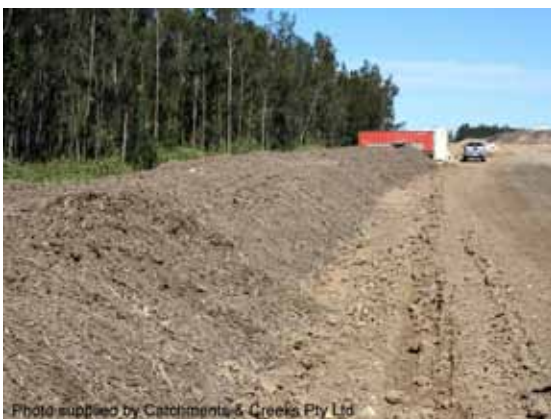
Mulch berm sediment control measure
