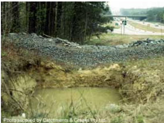
Excavated sediment trap
