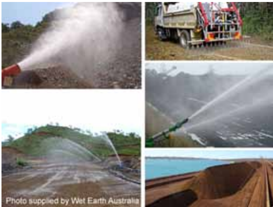
Application of soil binders
