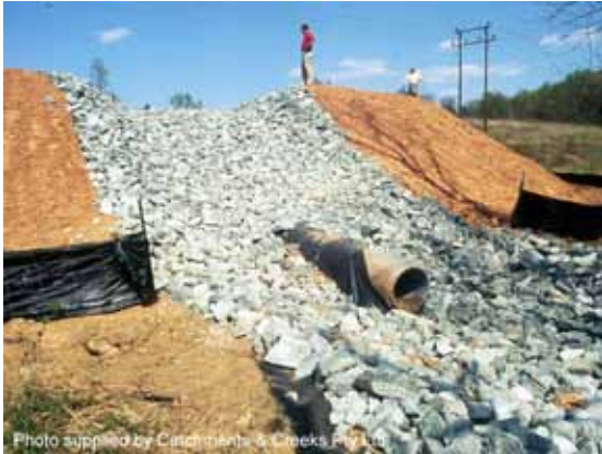
Spillway formed with fill embankment
