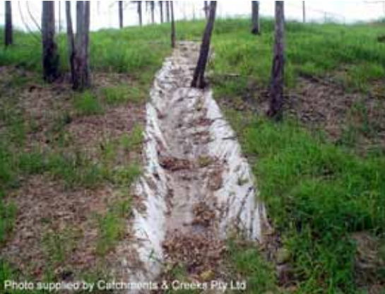
Geotextile lined drainage chute
