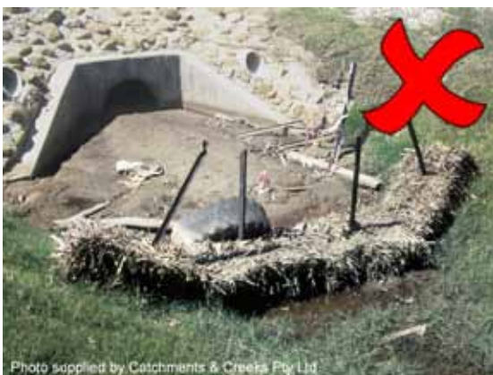
Inappropriate choice of sediment trap
