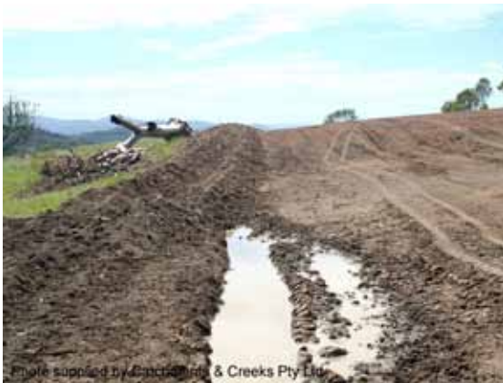
Flow diversion bank
