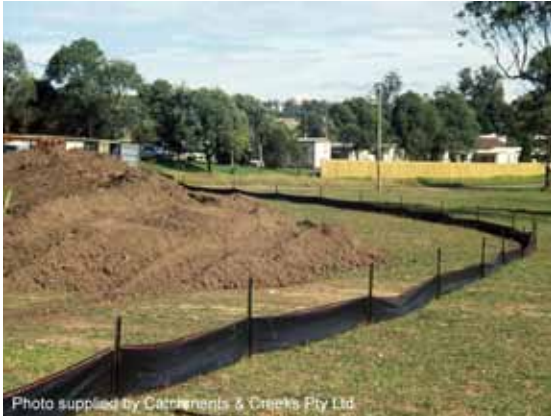
Stockpiling of topsoil
