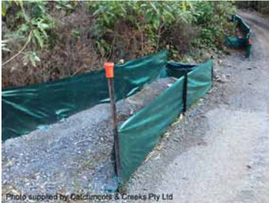
U-shaped sediment trap
