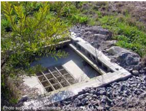
Block & aggregate drop inlet protection
