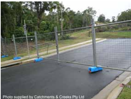
Temporary site fencing
