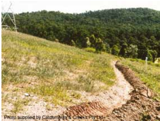
Earth-lined catch drain
