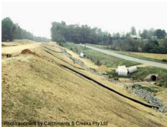
Slope drains on newly seeded batter
