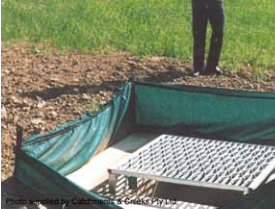
Fabric drop inlet protection
