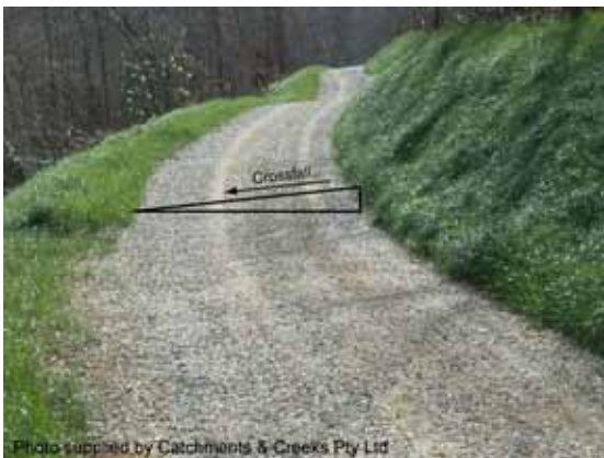
Gravel road with out-fall drainage
