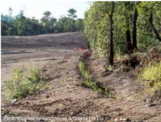
Flow diversion using a catch drain
