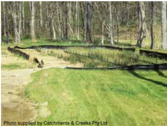
Coarse sediment trap
