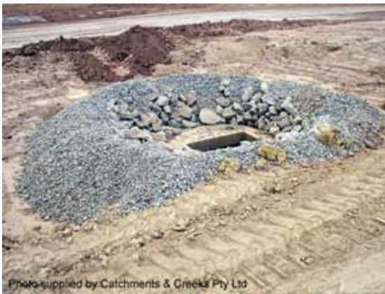
Rock & aggregate drop inlet protection
