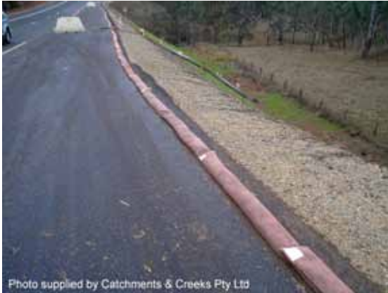
Sandbag flow control berm
