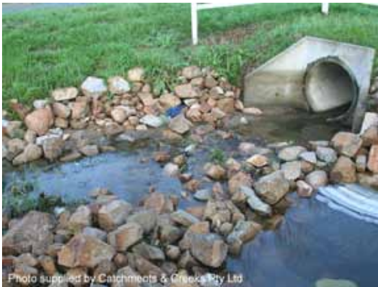
Rock pad outlet structure
