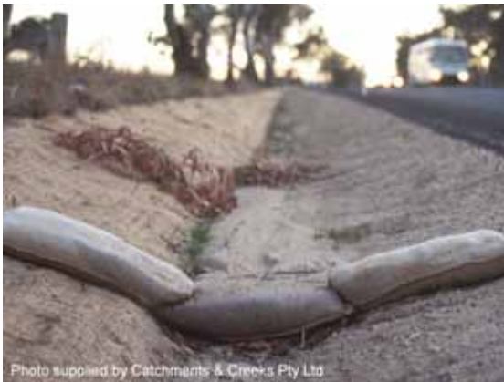
Sandbag check dam
