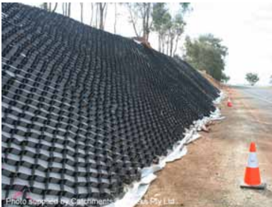
Installation on road batter
