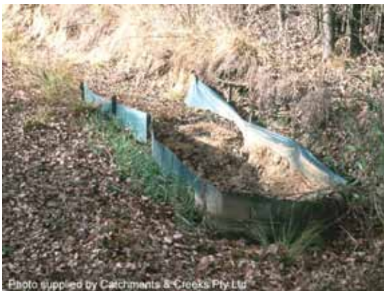
U-shaped sediment trap in steep drain
