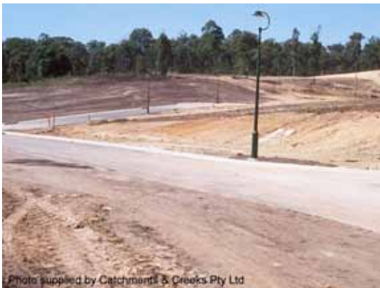
Replacement of topsoil
