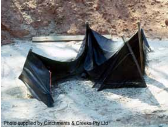
Storm damage to sediment trap
