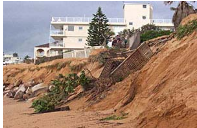
Erosion at Collaroy
