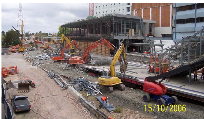
Chatswood Transport Interchange
