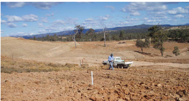
Doughboy hollow following soil conservation earthworks (diversion, shaping and filling)
