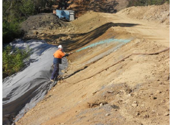
Soil polymer 'Gluon' being applied to exposed soil prior to rainfall
