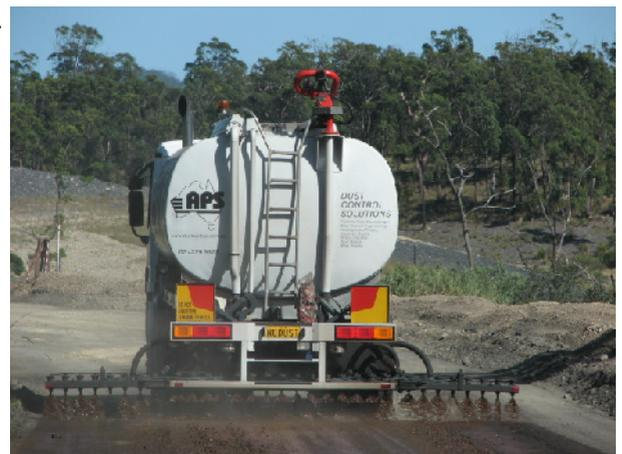
Bitumen based geobinder 'PetroTac' being applied to a mining haul road
