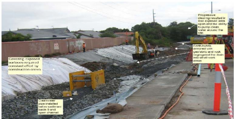
Figure 2. Construction of the 'triple-stack' design. Progressive clearing, segmentation, surface protection and clean water pipe construction.
