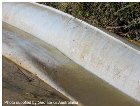
Photo 2 – A filter tube is just another form of filter bag
