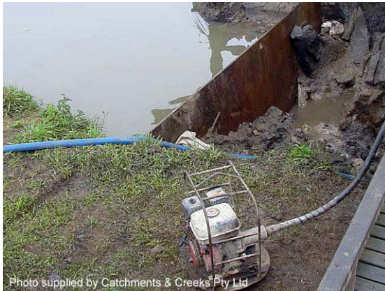
Photo 1 – De-watering an isolated work area
