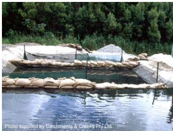
Photo 18 - Settling pond
