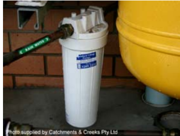
Photo 7 - Cartridge filter
