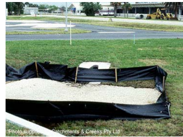
Photo 14 - Infiltration bed (permanent installation)
