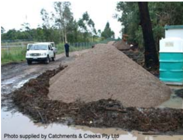
Photo 9 - Filter berm
