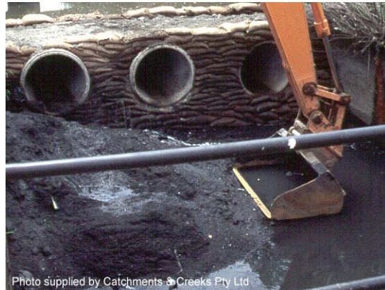
Photo 2 – De-watering of sediment prior to removal from a stormwater drain
