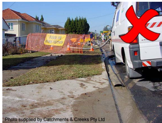
Photo 5 – De-watering should not discharge untreated into drains
