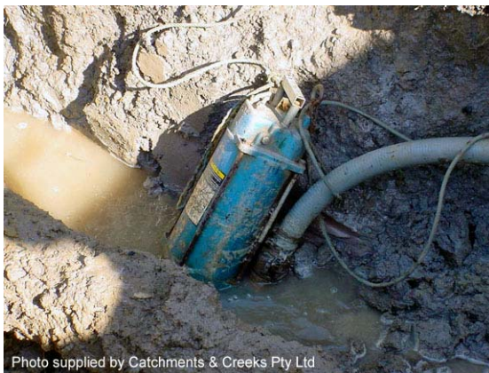
Photo 4 – Submersible pump de-watering an excavation
