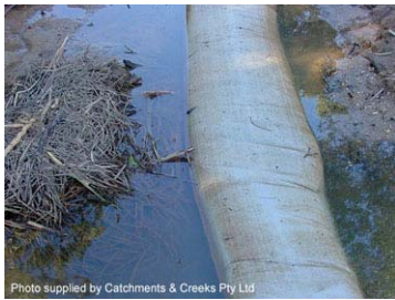
Photo 12 - Filter tube
