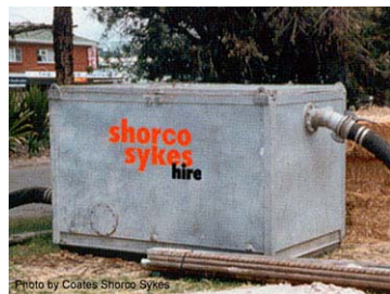
Photo 16 - Portable sedimentation tanks
