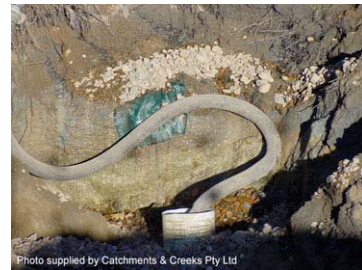
Photo 20 - Sump pit showing de-watering pipe exiting from the stand pipe
