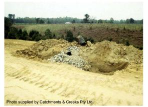
Photo 5 – Inlet sediment trap
