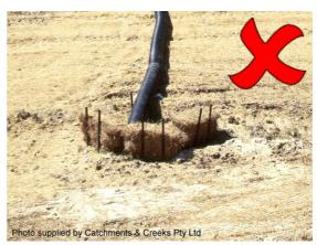
Photo 10 – Inappropriate flow release
