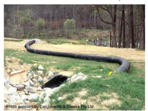
Photo 7 – Pipe directing flow to a sediment basin
