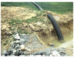
Photo 8 – Outlet sediment trap
