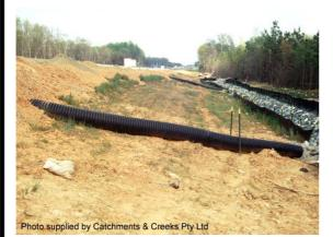
Photo 1 – Flexible, plastic slope drain
