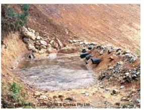
Photo 4 – Slope drains (right) used as an outlet structure for a sediment trap
