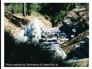
Photo 3 – Rock gabion and mattress channel stabilisation (during construction)
