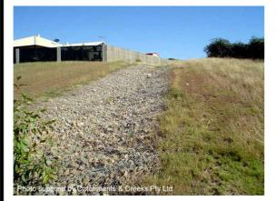
Photo 1 – Rock mattress-lined drainage chute
