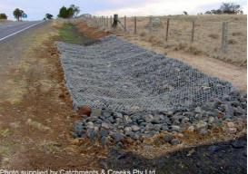
Photo 2 – Rock mattress-lined table drain (stormwater infiltration pit)
