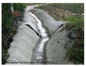
Photo 2 - Concrete lined catch drain
