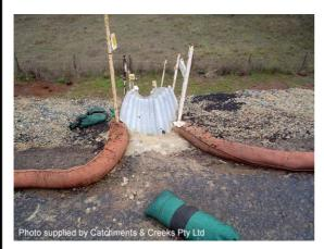
Photo 1 – Batter chute formed from corrugated sheet iron
