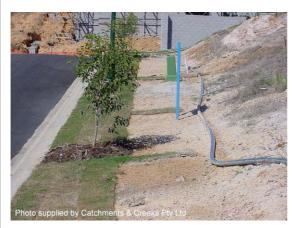
Photo 5 – Lateral turf strips can reduce the risk of flow diversion along up-slope edge of turf
