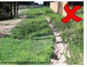
Photo 4 – Undesirable rilling along edge of turf caused by lateral inflows
