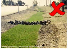
Photo 8 – Check dams and sediment traps placed on turfed drains can cause flow bypassing and erosion (rilling) along the edge of the turf
