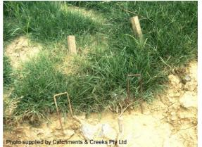
Photo 6 – Turf should be anchored with wooden pegs, not metal staples
