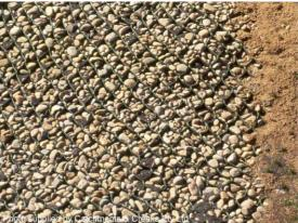
Photo 2 – Cellular confinement system integrated with rock mulching used as a form of erosion control
