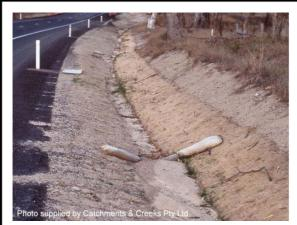
Photo 3 – Check dam sediment trap
