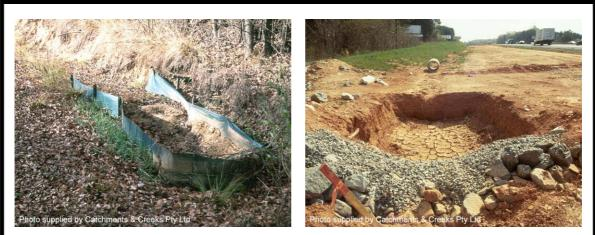
Photo 1 – U-shaped sediment trap
