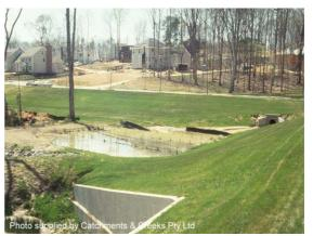
Photo 10 – Example of various purposedesign stormwater outlet sediment traps
