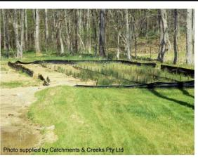
Photo 4 – Coarse sediment trap
