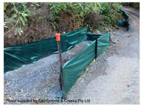
Photo 9 - U-shaped sediment trap
