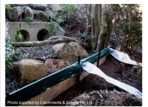
Photo 5 - Filter tube dam
