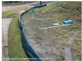
Photo 1 - Sediment-laden sheet flow
