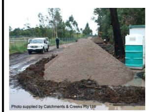
Photo 3 – Smaller berms are best formed from composted material
