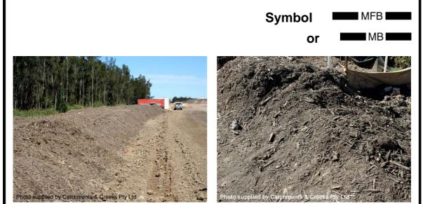
Photo 1 – Large mulch filter berm
