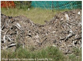
Photo 4 – Mulch filter berms need to be sufficiently large (high) to allow for possible slumping and damage by foot traffic
