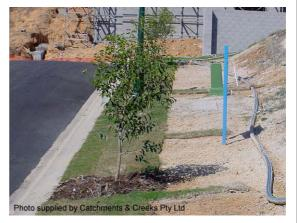
Photo 6 – Example of grass filter strips with lateral turf strips used to reduce the risk of rilling along the up-slope edge of the turf
