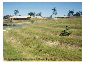
Photo 3 – Grass filter strips placed along the contour
