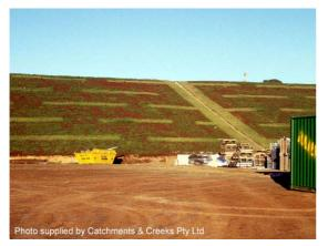
Photo 1 – Grass filter strips placed on a newly vegetated slope
