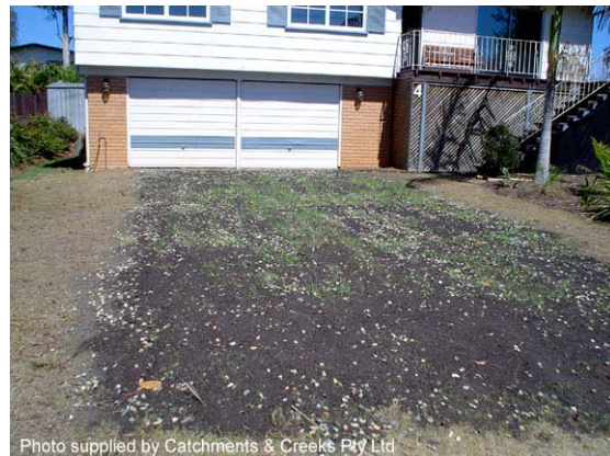
Photo 2 – Stage 1: fill voids with soil, then seed (non-traffic period)
