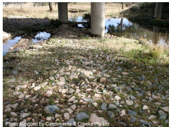
Photo 4 – Grassed structural soil used for erosion control under a rural bridge
