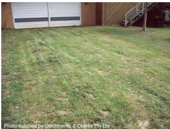
Photo 3 – Stage 1: Establishment of grassed surface (vehicular traffic allowed)
