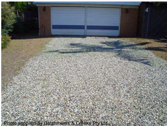
Photo 1 – Stage 1: placement of aggregate
