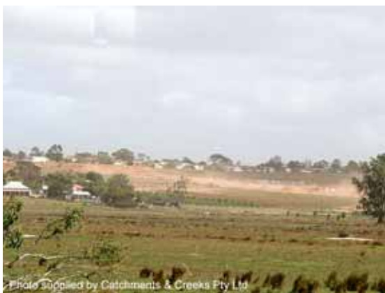
Photo 1 – Dust generation on a construction site
