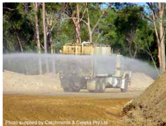
Photo 2 – Dust control using a water truck
