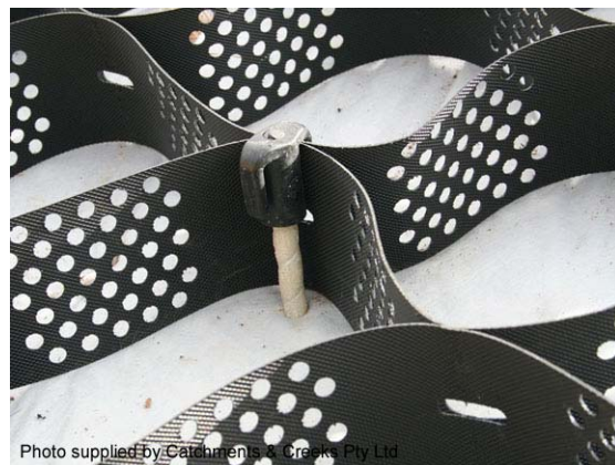
Photo 28 – Cellular confinement system
