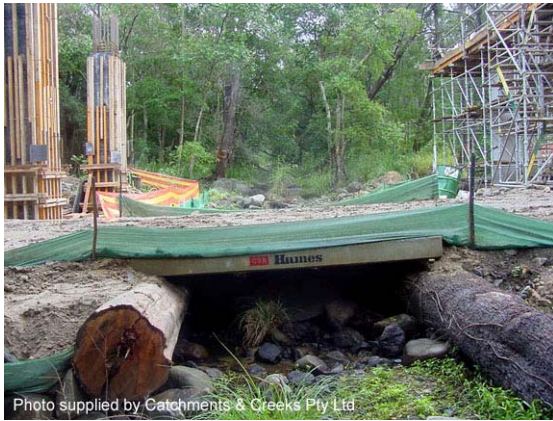
Photo 21 – Temporary bridge crossing
