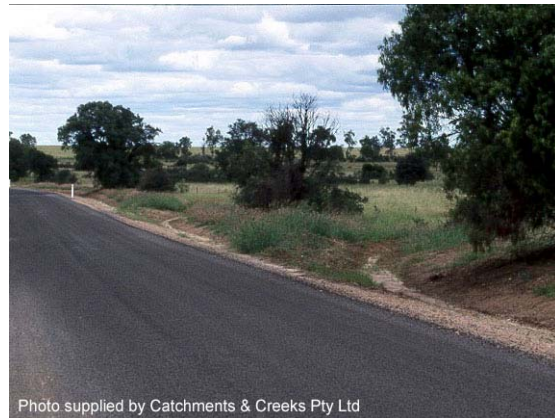
Photo 18 – Several diversion drains on a sealed roadway
