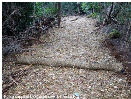
Photo 30 – Fibre rolls used to control drainage during track rehabilitation
