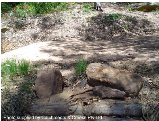
Photo 11 – Cross-bank showing discharge structure (foreground)
