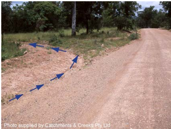
Photo 17 – Diversion drain on an unsealed rural road
