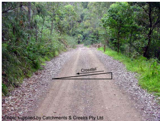
Photo 5 – Example of 'infall' road crossfall
