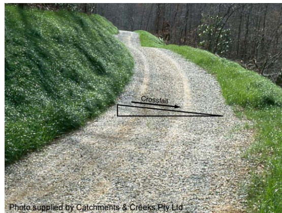
Photo 6 – Example of 'outfall' road crossfall
