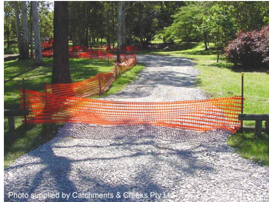
Photo 2 – Temporary construction access road through parkland
