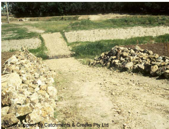
Photo 23 – Temporary ford crossing
