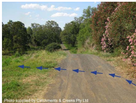
Photo 20 – Flow diversion cross bank (difficult to see in photo) just prior to the road falling to a creek crossing
