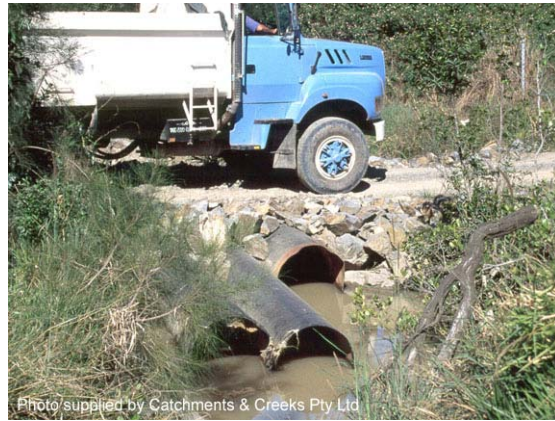
Photo 22 – Temporary culvert crossing
