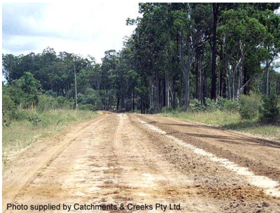
Photo 31 – Grading of fines in towards the centre of the road before re-profiling
