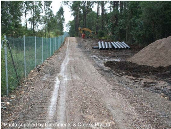
Photo 1 – Permanent construction and maintenance access road
