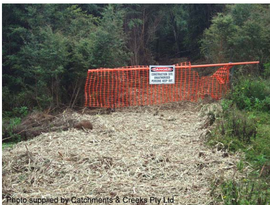
Photo 29 – Rehabilitation of access track
