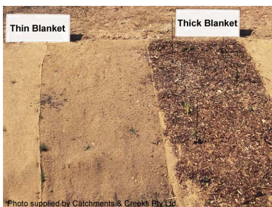
Photo 27 – Erosion control blankets
