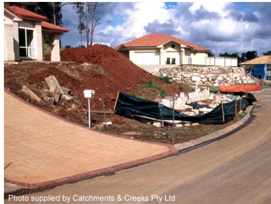
Photo 34 – Sediment barriers must not extend onto the road verge unless appropriate approval is obtained
