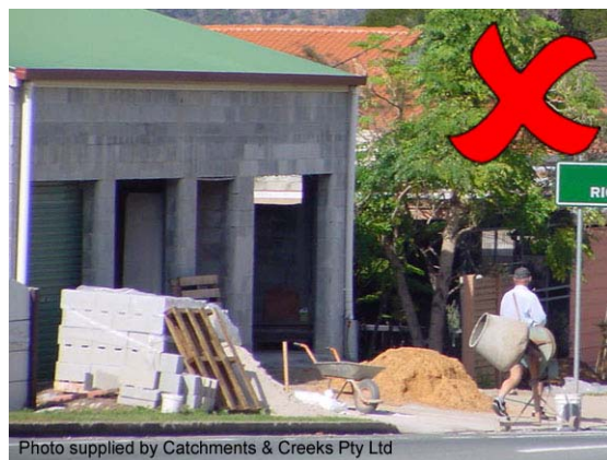
Photo 36 – Building works should not occur on the road verge
