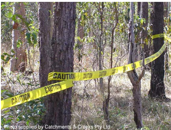
Photo 5 – Caution tape used to identify non-disturbance areas and protected vegetation
