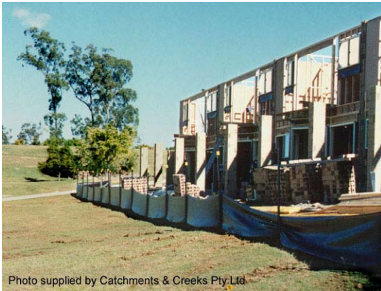
Photo 21 – Sediment fence placed along the contour down-slope of a building site
