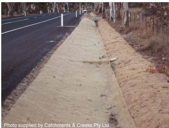
Photo 13 – Stormwater drain lined with a 'jute' erosion control mat
