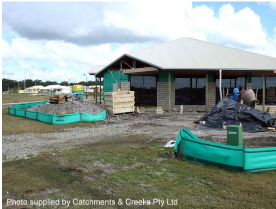
Photo 9 – Note earth stockpile behind sediment fence (left), and covered stockpile (right)
