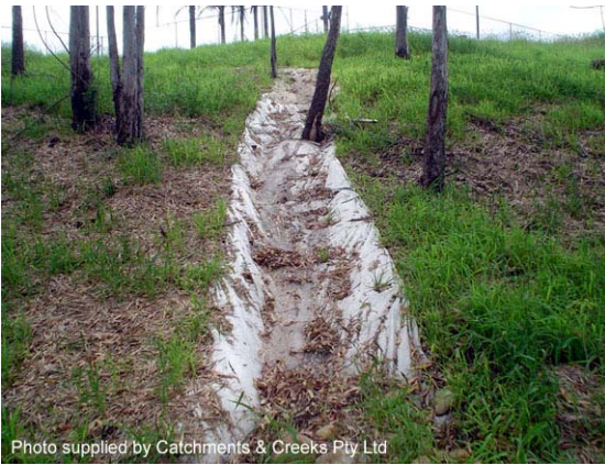
Photo 17 – Geotextile filter cloth used as a temporary lining within a chute
