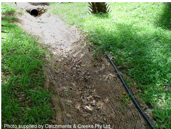
Photo 15 – Stormwater drain lined with jute mesh
