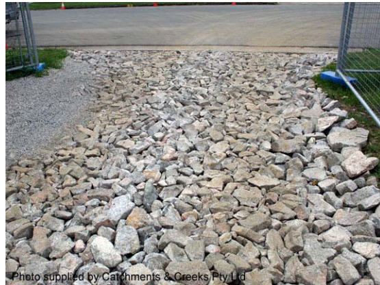
Photo 8 – Rock pad showing use of large, uniform rock
