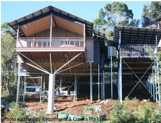
Photo 3 – Steep sites require appropriate building design
