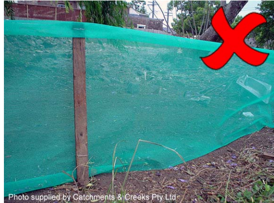
Photo 24 – Shade cloth must NOT be used to form a sediment fence
