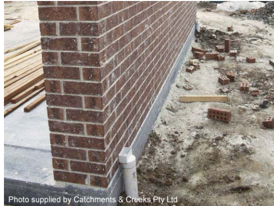
Photo 30 – Installation of permanent drainage system before roof framing
