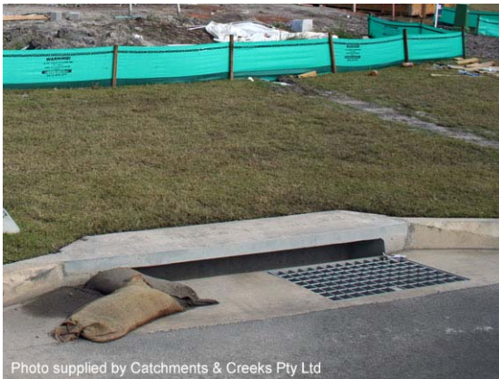
Photo 33 – Sediment barriers must only be placed within the road reserve upon the approval of the road authority
