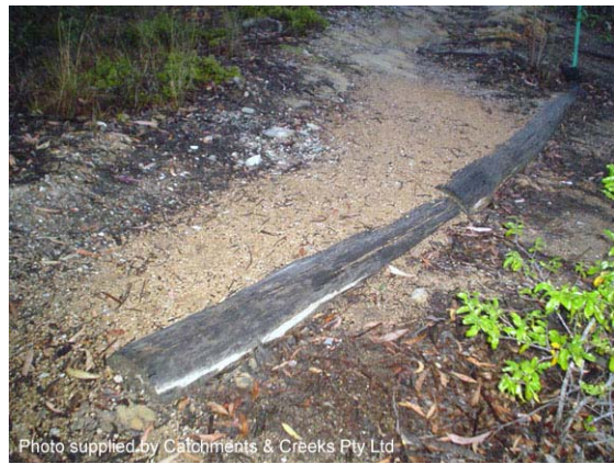
Photo 18 – Recessed log used as a level spreader to release runoff as 'sheet' flow
