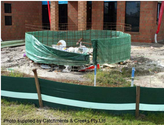
Photo 31 – Site rubbish pit protected from wind through the use of a ‘sediment fence’ wind break
