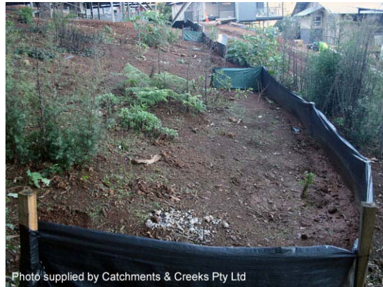
Photo 22 – Sediment fence showing use of regular 'returns'
