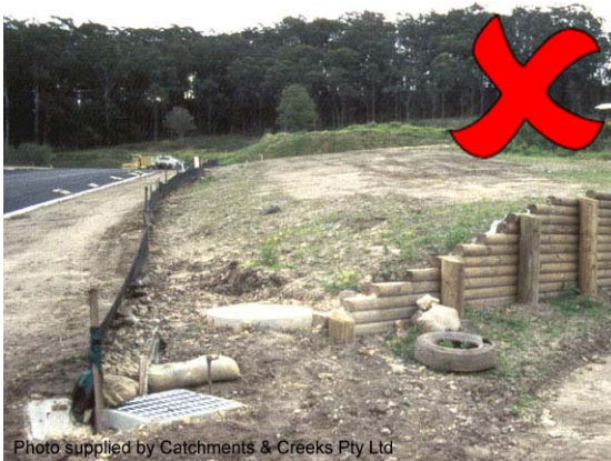
Photo 23 – Poorly installed sediment fence directing sediment-laden runoff directly into a stormwater inlet
