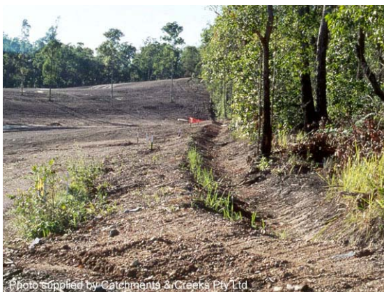
Photo 11 – Catch drain up-slope of a soil disturbance
