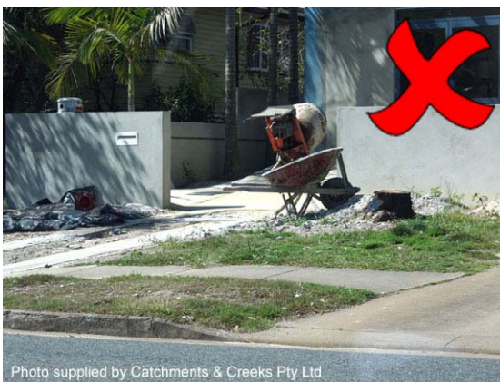
Photo 35 – Building works should not occur on the road verge
