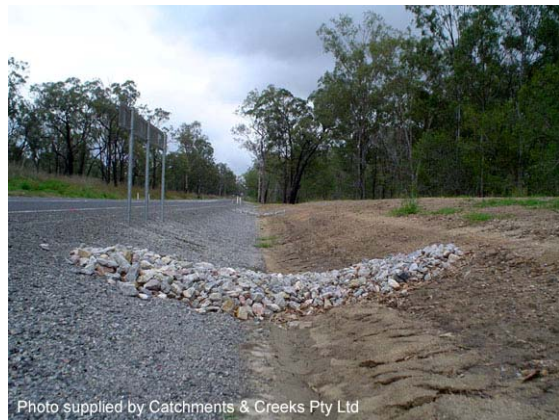
Photo 20 – Rock check dam used to reduce flow velocities in drains
