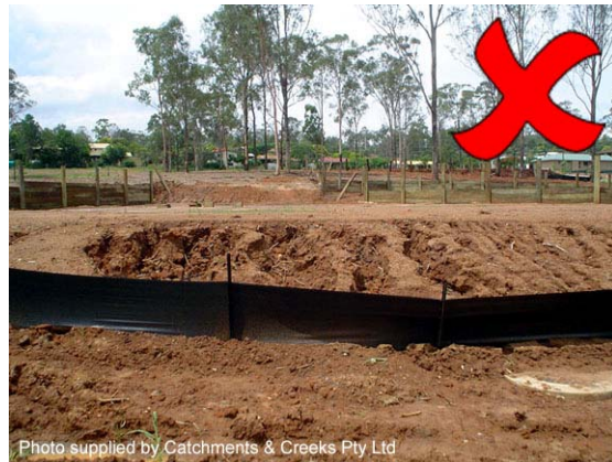
Photo 4 – Poor soils can result in erosion problems even before building works start
