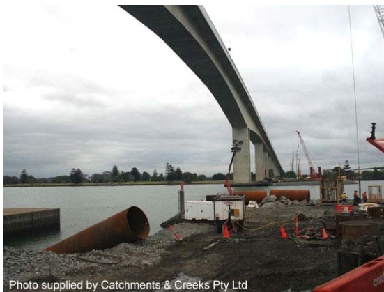
Photo 5 – Construction works isolated from river flows through the use of land reclamation
