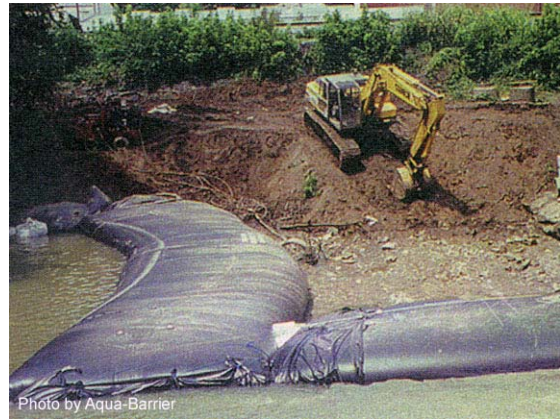
Photo 2 – Isolation barrier formed from water-filled rubber dams
