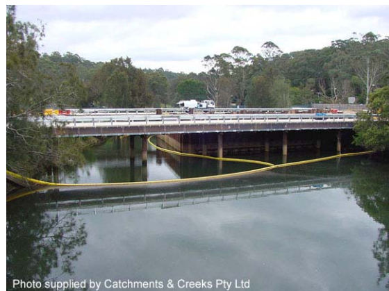
Photo 6 – Isolation barrier formed from sheet piling
