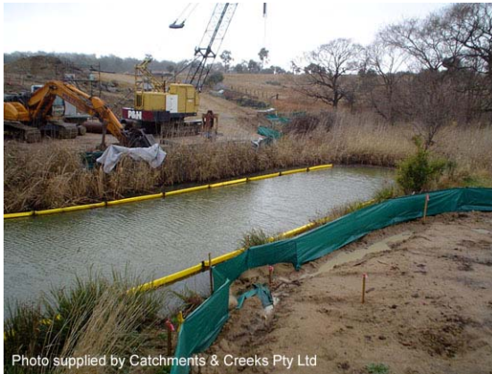
Photo 1 – Isolation barriers formed from silt curtain
