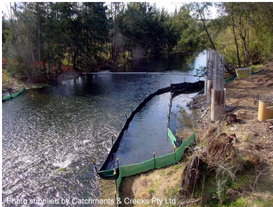
Photo 3 – Isolation barrier formed from sediment fence fabric
