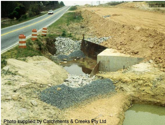
Photo 11 – Excavated sediment trap associated with culvert construction
