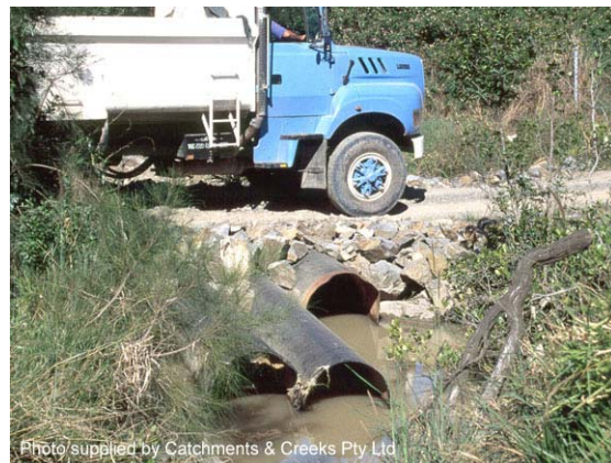
Photo 8 – Temporary culvert crossing
