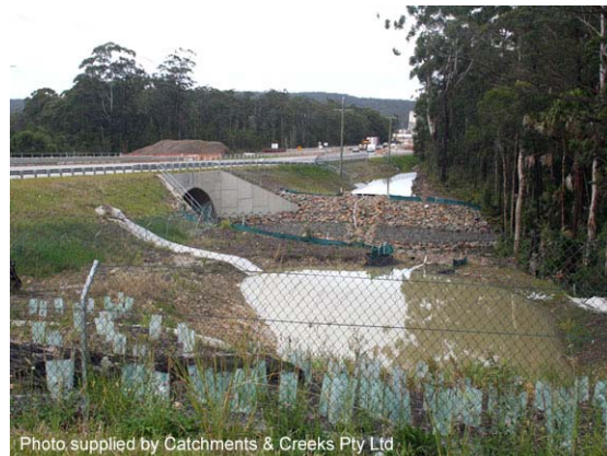
Photo 14 – Construction sediment basins retained as permanent stormwater treatment ponds
