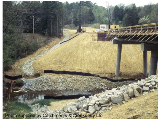
Photo 12 – Bridge construction showing one of four rock filter dam sediment traps
