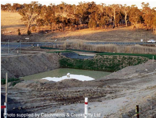
Figure 13 – Sediment basin adjacent a new culvert crossing
