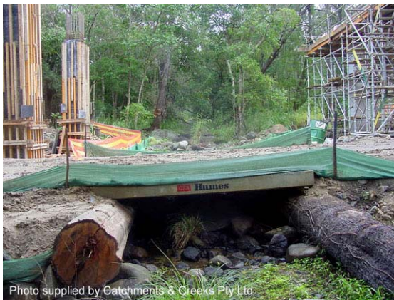
Photo 7 – Temporary bridge crossing
