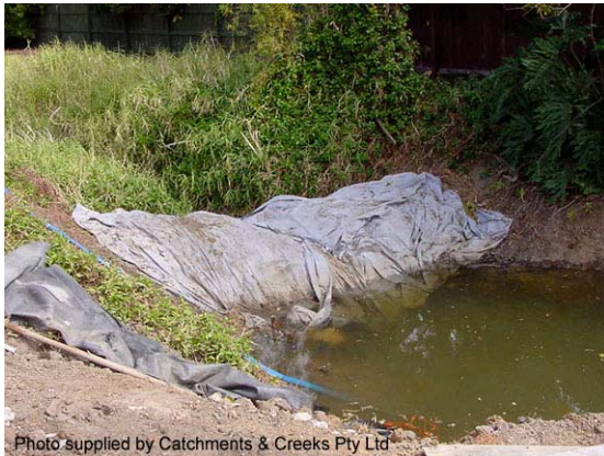
Photo 3 – Rock filter dam
