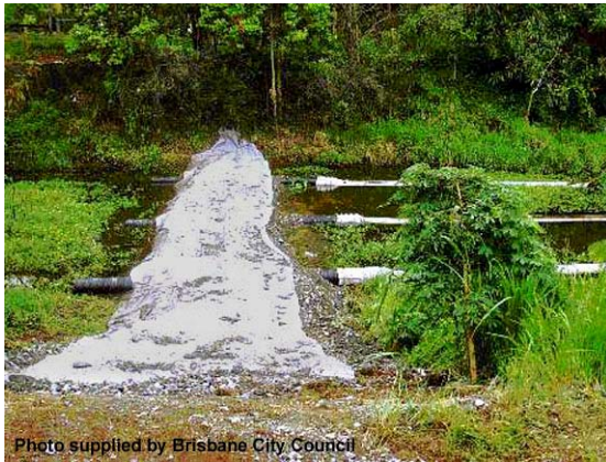
Photo 1 – Filter tube barrier
