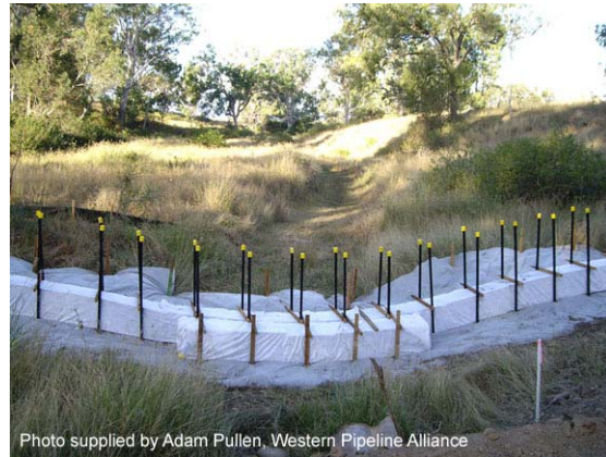
Photo 2 – Modular sediment barrier
