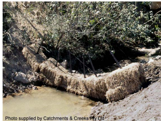
Photo 6 – Straw bale barrier
