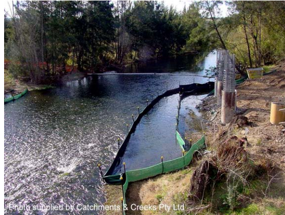
Photo 2 – Sediment fence isolation barrier
