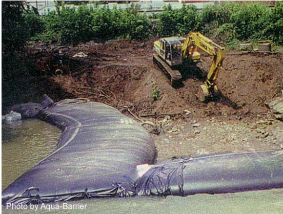
Photo 1 – 'Aqua Barrier' water-filled isolation barrier
