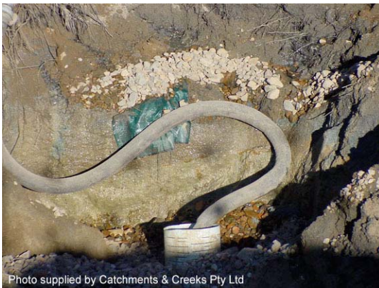
Photo 1 – Sump pit in operation
