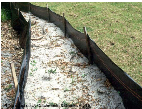
Photo 1 – A sediment fence can be used to spread inflows evenly across the full width of the grassed filter bed
