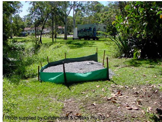
Photo 2 – Combined aggregate and filter fence sediment control system
