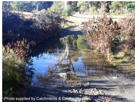
Photo 2 – Ford crossing of alluvial (gravel) stream
