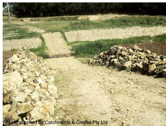
Photo 6 – Ford crossing of newly constructed stormwater drain
