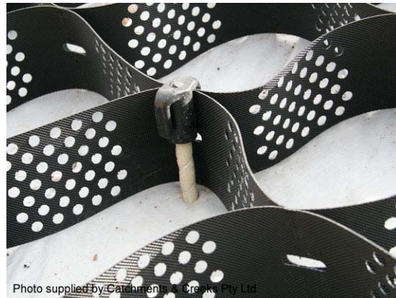
Photo 4 – Cellular confinement system
