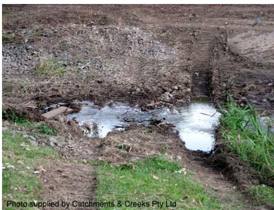
Photo 5 – Temporary gravel-stabilised ford crossing of clay-based creek
