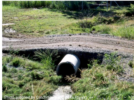
Photo 2 – Temporary crossing of minor drainage channel
