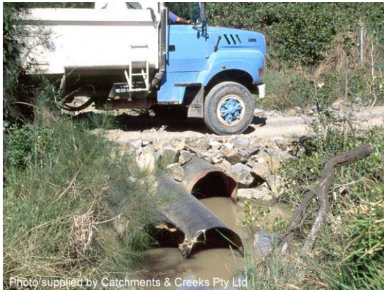
Photo 1 – Temporary culvert formed from recycled steel pipes
