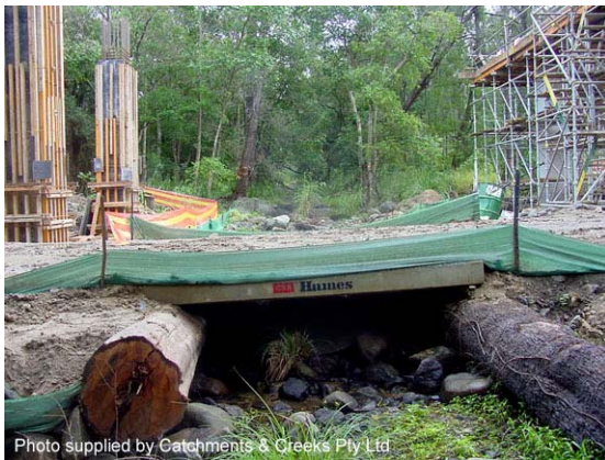
Photo 1 – Temporary bridge crossings formed with a 'culvert bridging slab'
