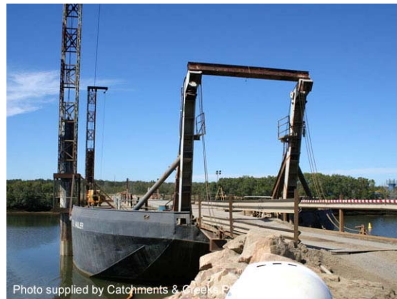
Photo 2 – A barge used for the temporary crossing of tidal watercourse
