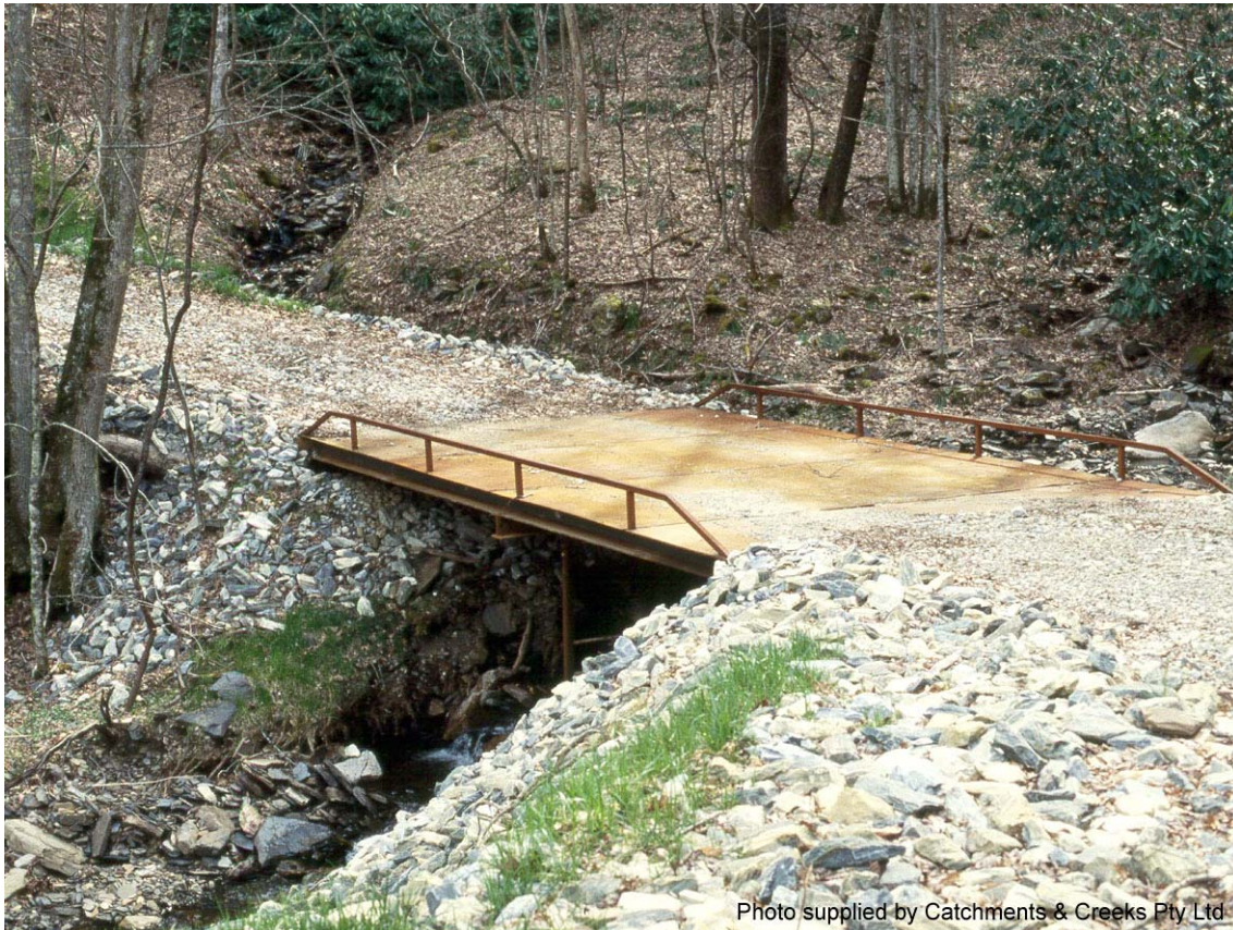
Photo 3 – Temporary steel deck bridge on a construction access road
