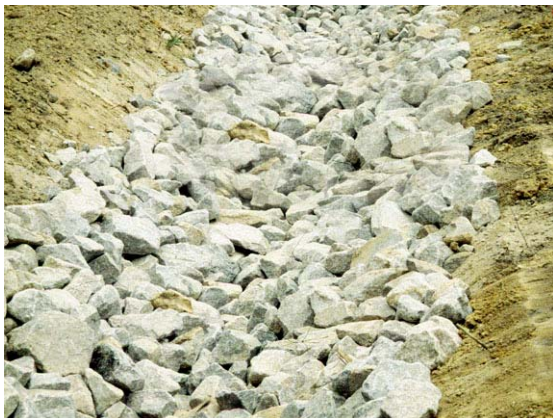
Photo 5 – Placement of the rock on the soil can result in erosion problems if significant lateral inflows occur
