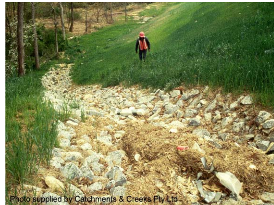
Photo 2 – Permanent, rock-lined batter chute
