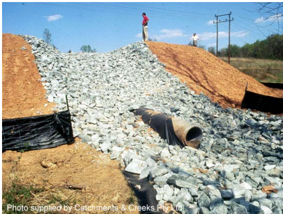
Photo 1 – Rock-lined emergency spillway of a sediment basin
