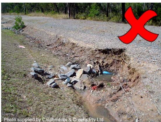
Photo 9 – Typical erosion problem when placed in dispersive soil
