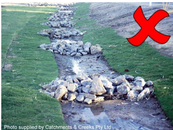
Photo 7 – Poor placement of rocks, note rocks are higher in centre of check dam
