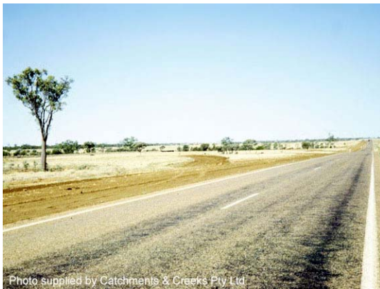
Photo 1 – Diversion drains (centre) collect stormwater from roadside table drains, then releases the water as sheet flow via a level spreader
