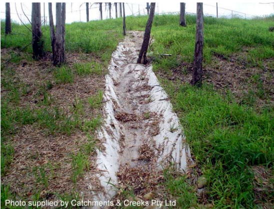
Photo 1 – Temporary chute lined with filter cloth
