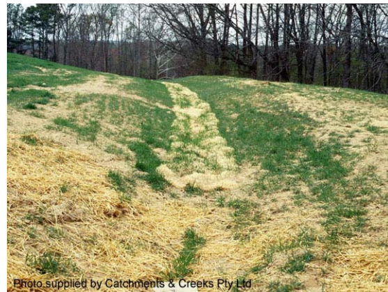
Photo 2 – Diversion drain lined with composite wood shaving mat
