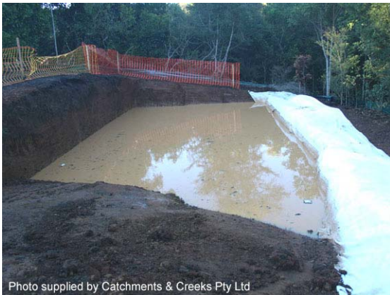
Photo 5 – Recessing the basin into the ground allows the natural ground level to become the spillway
