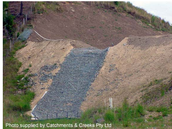
Photo 2 – Rock mattress-lined sediment basin emergency spillway
