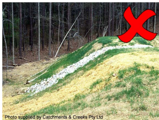
Photo 8 – A suitable energy dissipater must exist at the base of the spillway
