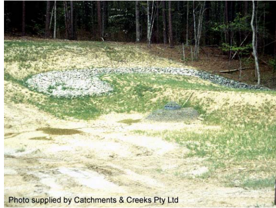
Photo 4 – Rock-lined spillway cut into virgin soil (note the spillway is curved up to the crest, after which it remains straight)
