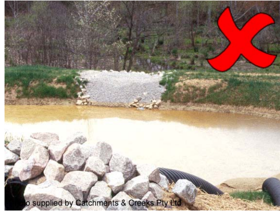
Photo 20 – Rock-lined spillway with poorly defined crest profile
