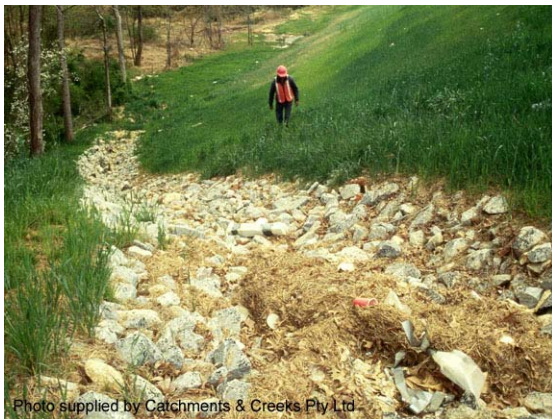
Photo 17 – Permanent, rock-lined batter chute
