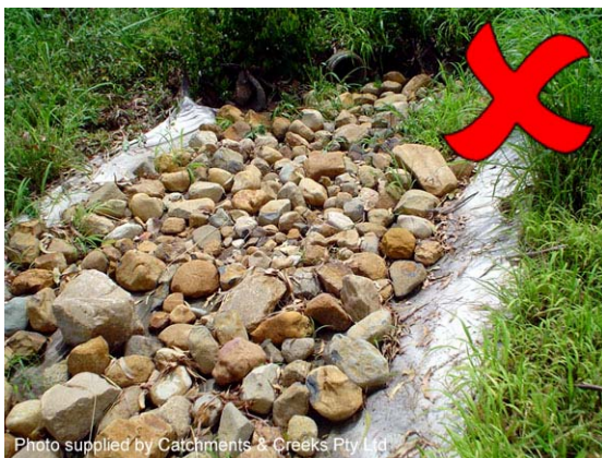
Photo 23 – Rounded rock can be significantly less stable than angular, fractured rock, especially when placed on steep slopes
