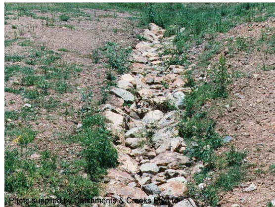
Photo 18 – Permanent, rock-lined batter chute
