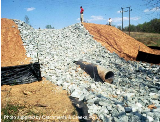
Photo 19 – Rock-lined spillway with well-defined crest profile
