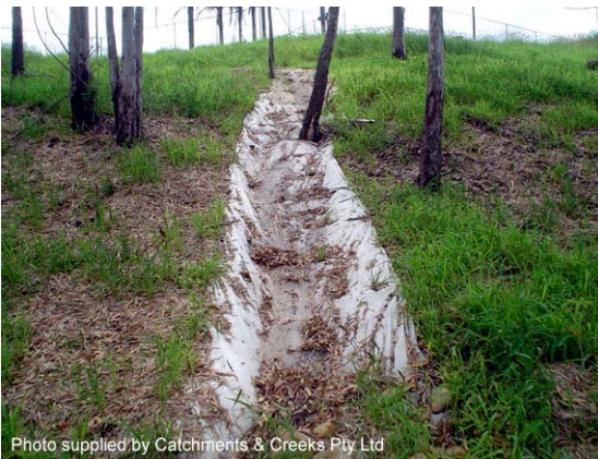
Photo 9 – Temporary chute lined with filter cloth
