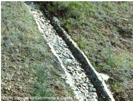
Photo 1 – Permanent, grouted-stone batter chute
