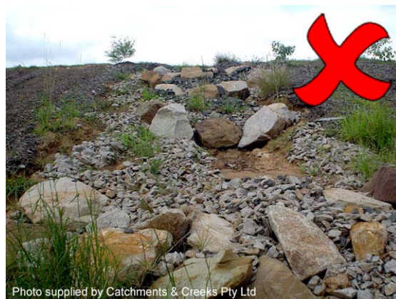
Photo 8 – Erosion caused by inadequate rock size and water bypassing around the poorly located boulders
