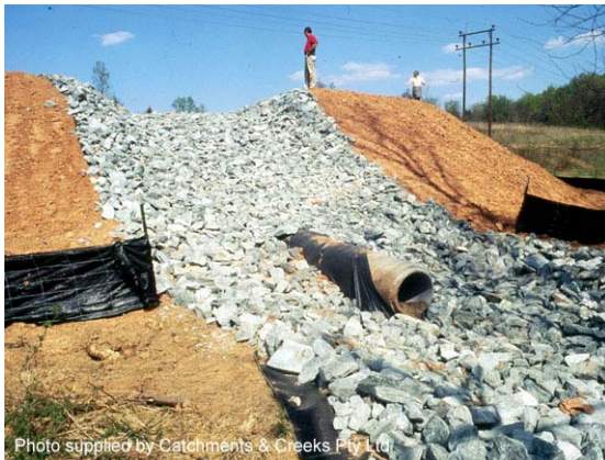
Photo 5 – Spillway chute with well-defined inlet profile
