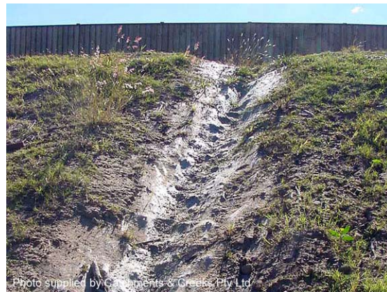
Photo 2 – Temporary batter chute lined with filter cloth
