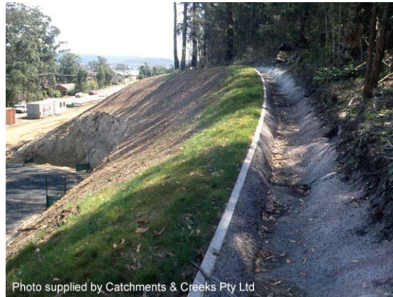
Photo 4 – Permanent catch drain
