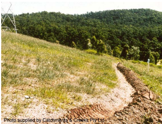
Photo 1 – Unlined catch drain
