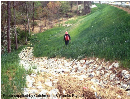
Photo 3 – Rock lined catch drain
