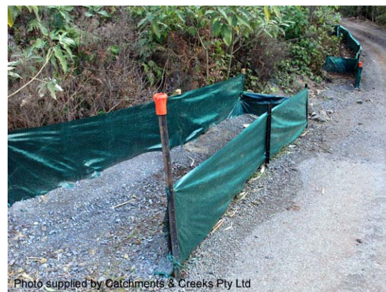
Photo 2 – U-shaped sediment trap within a mild gradient table drain
