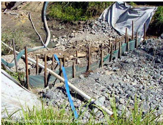
Photo 5 – Instream sediment weir with downstream splash pad
