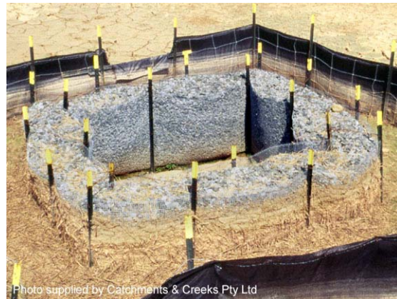
Photo 2 – Sediment weir used as a control structure around a filed (drop) inlet
