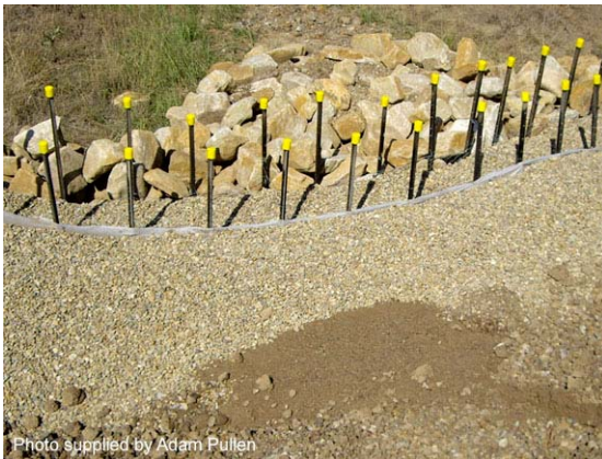
Photo 1 – Sediment weir (up-slope face) showing aggregate filter
