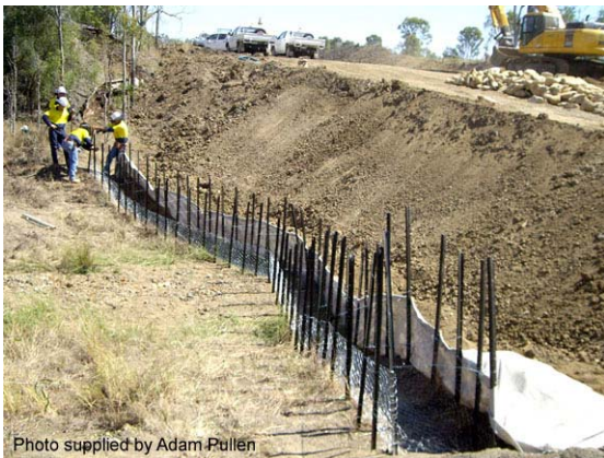
Photo 3 – Installation of an off-stream sediment weir
