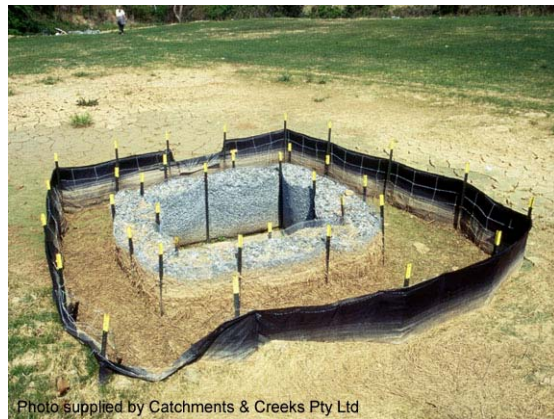
Photo 4 – Sediment weir used as a control structure around a field (drop) inlet
