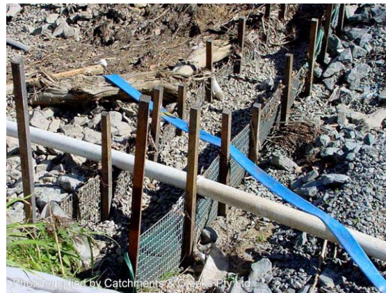
Photo 6 – Sediment weir (left) showing aggregate infill
